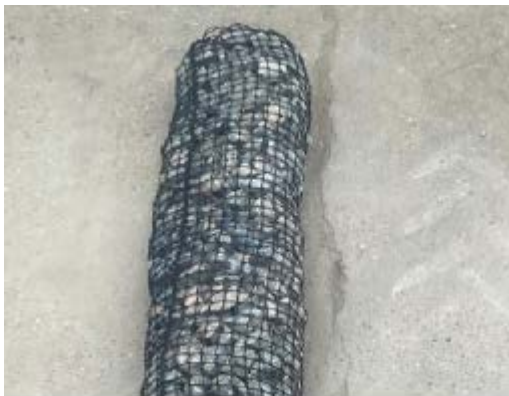
Fig 3: Typical Detail of Rock Roll
