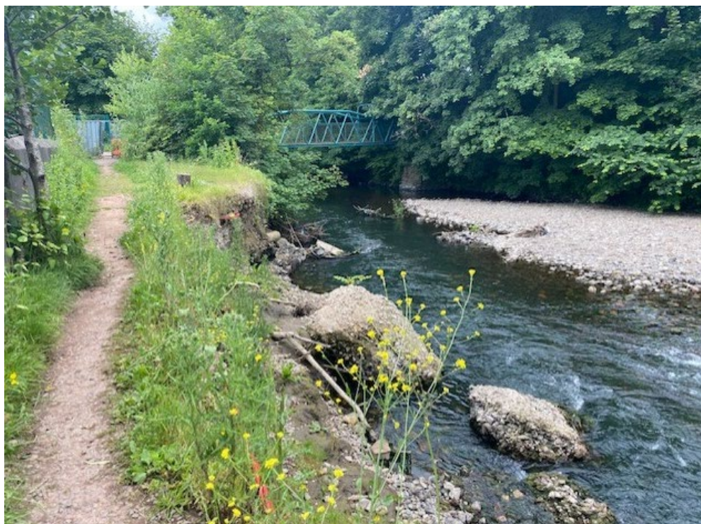
Site of river bank collapse looking south towards footbridge and illustrating pebble beach opposite
