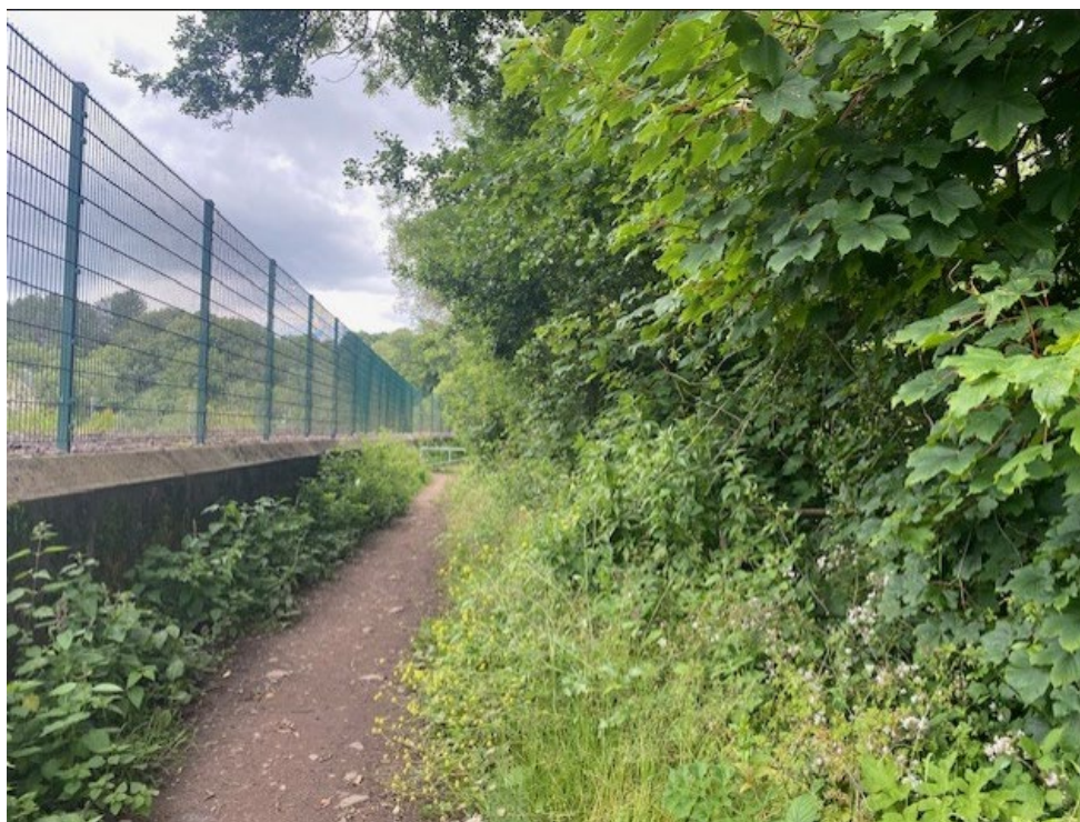
Path south of site illustrating likely vegetation structure that would have been present at the site before the collapse
