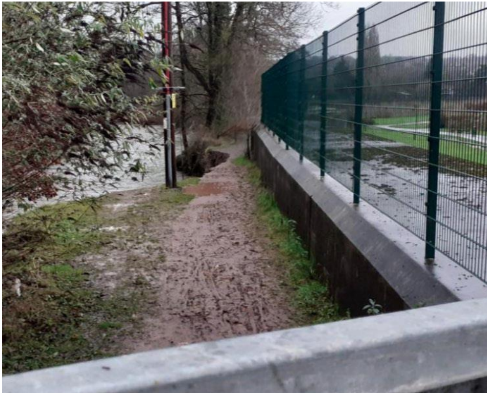
Photograph 4: View upstream from the footbridge along the flood wall
