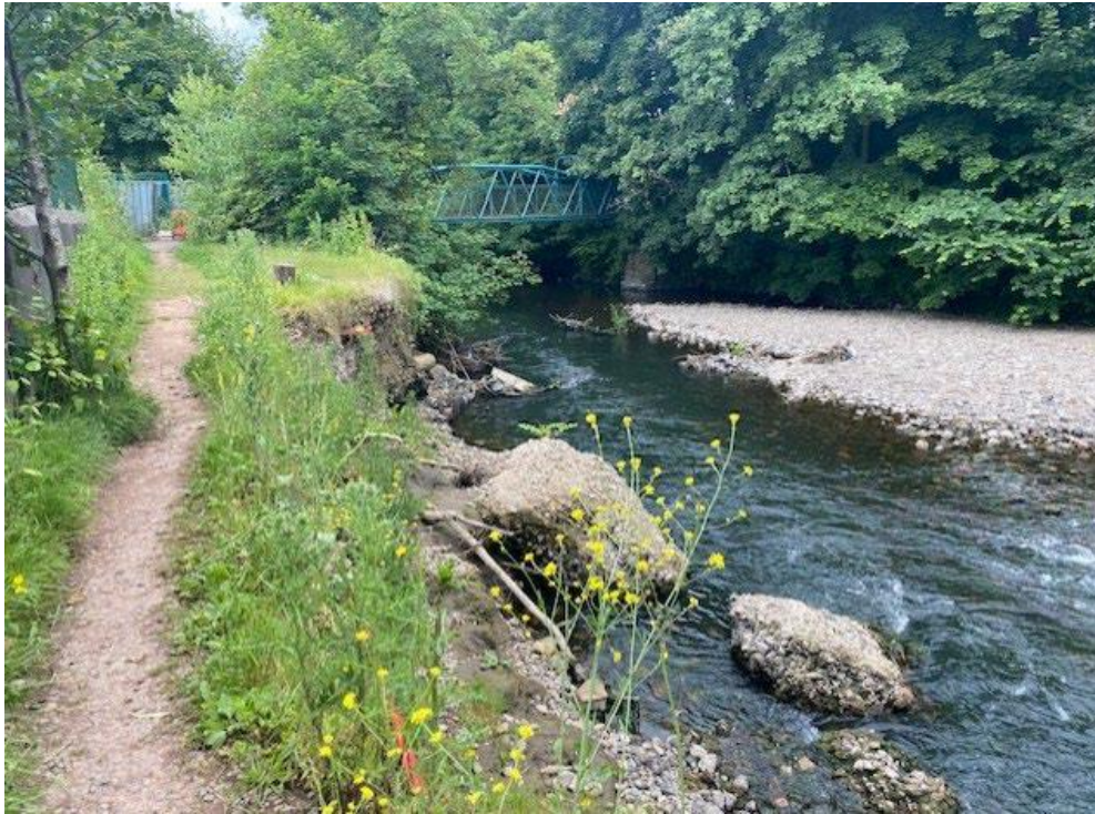
Photograph 5: View downstream towards the footbridge
