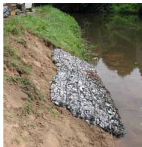
Rock Mattress placed on river bank
