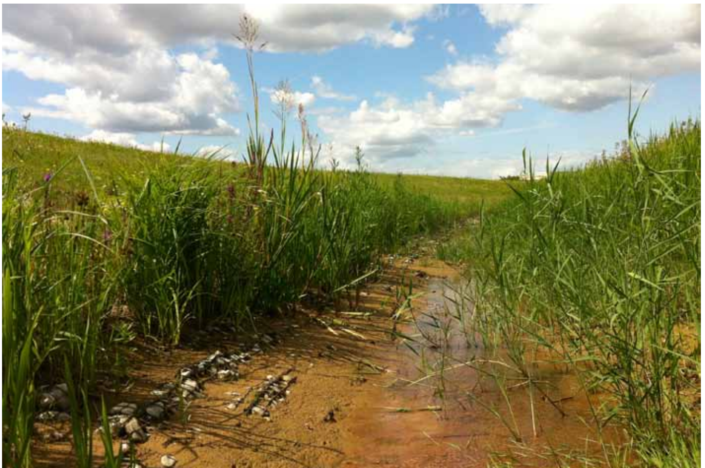
Recently installed Rock Mattresses at the base of a spillway accrete silt and allow vegetation establishment
