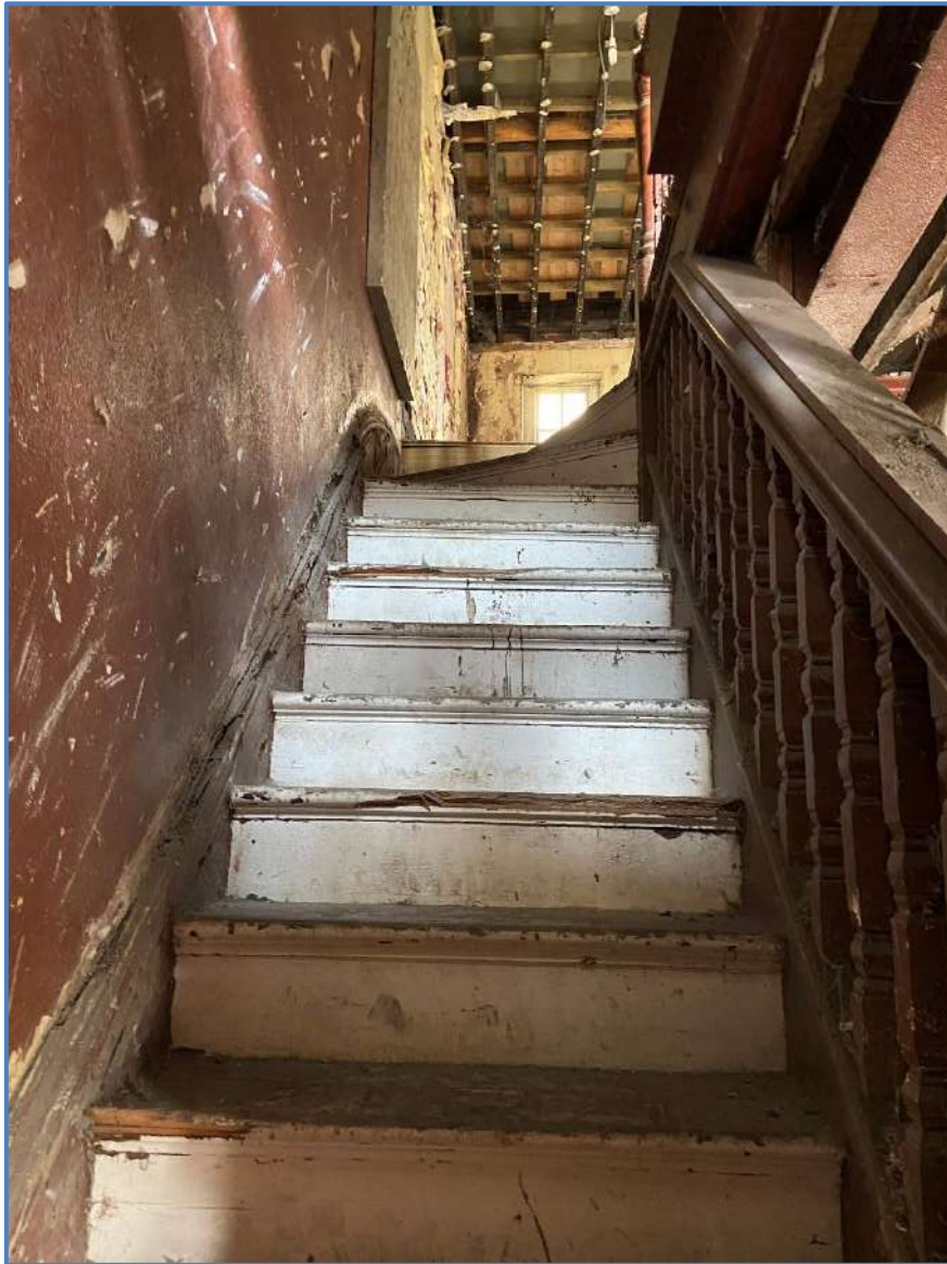
Images 32 and 33 – Details of the original staircase, going to the second floor.
