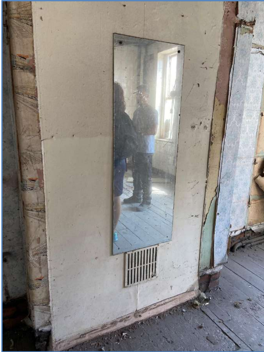
Images 52 and 53 – Second floor. Details of wall facing towards no.12 Clarence Place.
