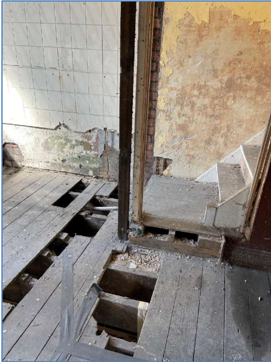
Images 54 and 55 – Second floor. Details of wall facing towards no.12 Clarence Place.
