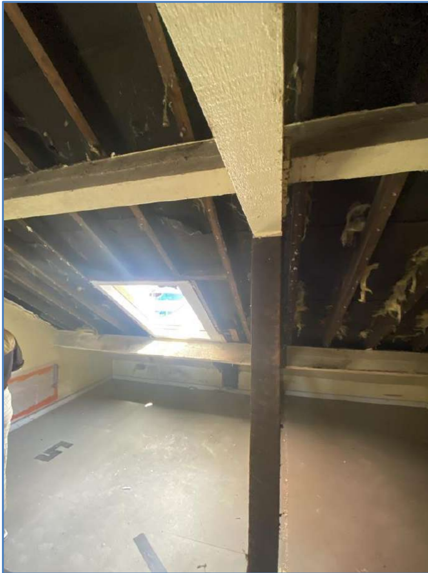
Images 59 and 60 – Third floor. Details of original rooflights.
