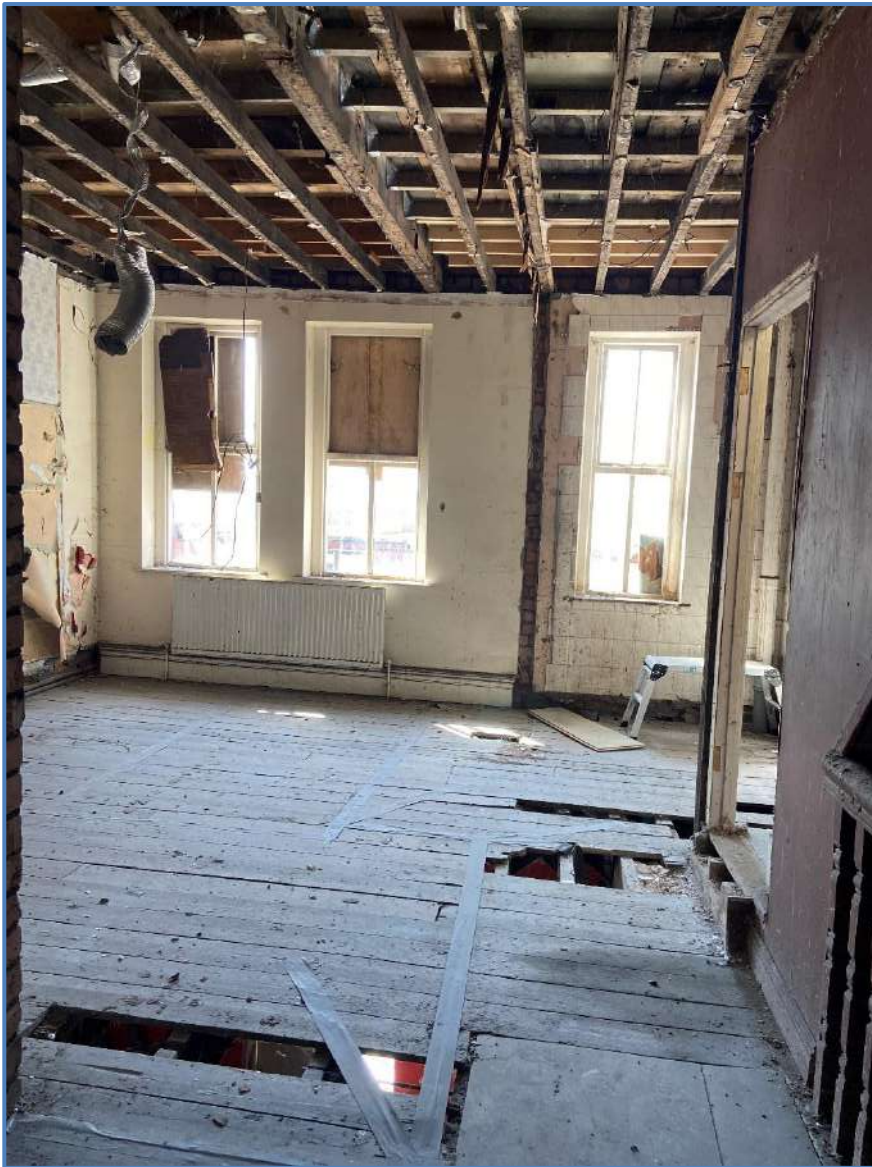
Images 46 and 47 – Second floor, looking towards the rear of the building.
