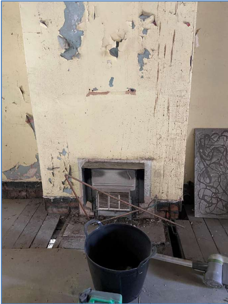
Images 44 and 45 – Second floor, details of the fireplace, which is not original.
