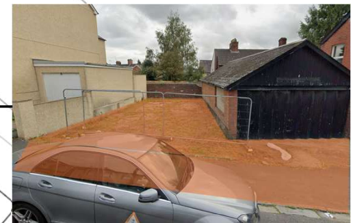
Construction laydown and parking area
