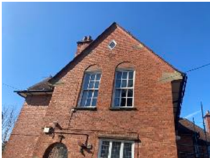
South east gable end of building
