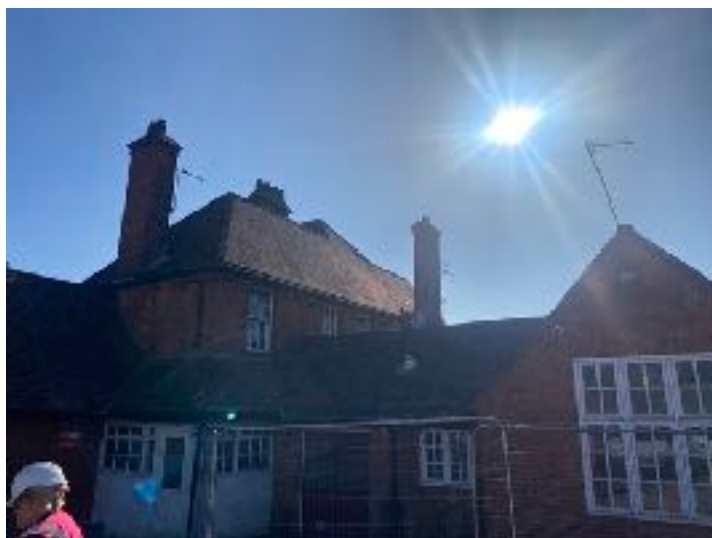
North elevation of building
