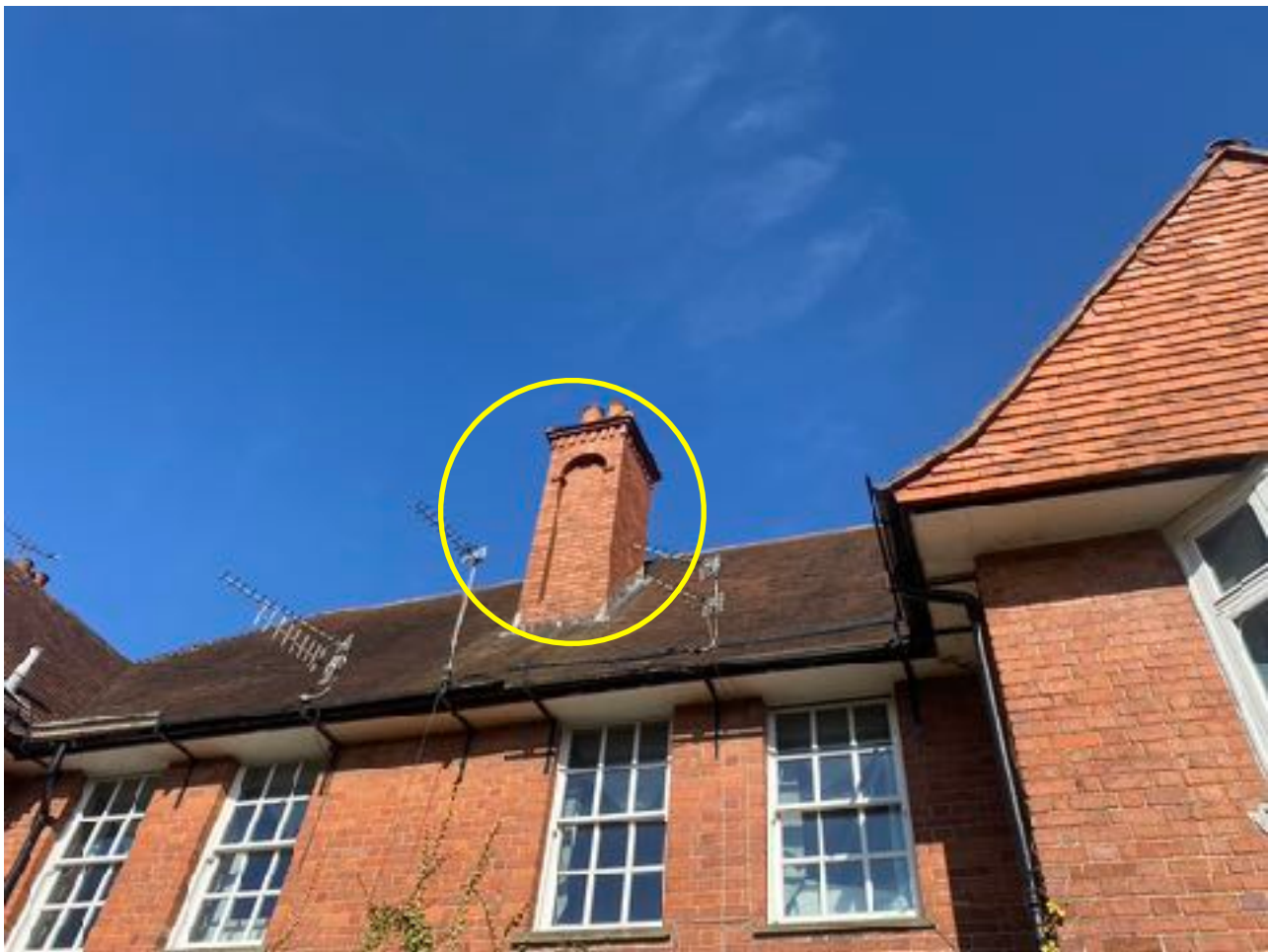
Chimney on south west pitch of roof - bat box location
