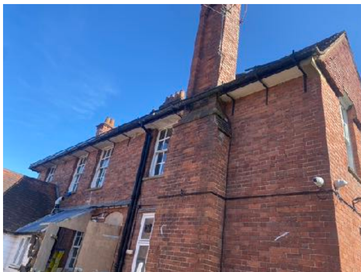
North west elevation of building
