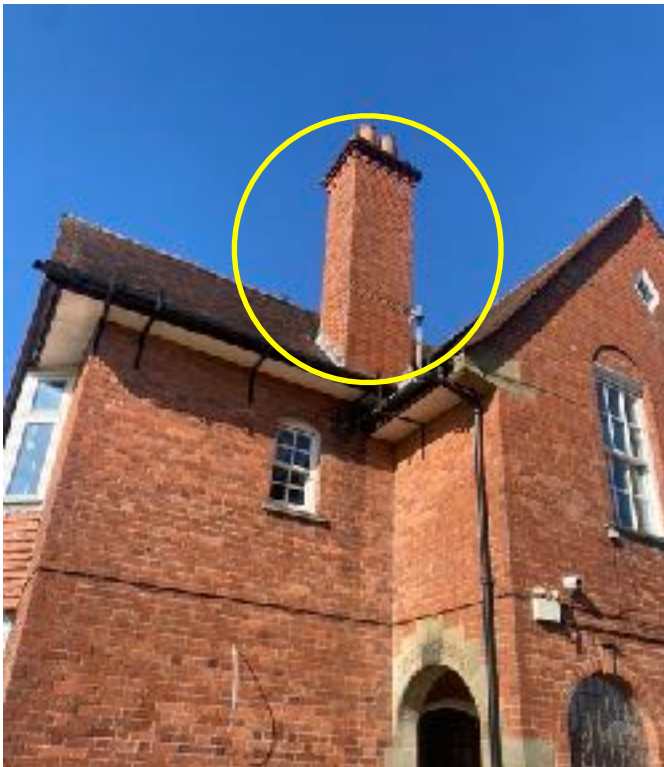
Chimney to south east of roof - bat box location
