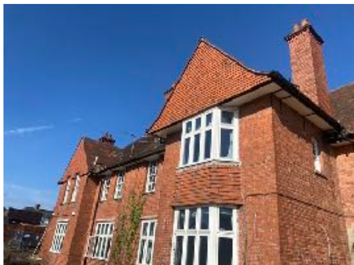
South west elevation of building
