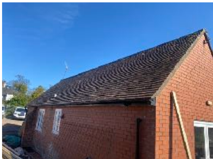
North west elevation of single story section of building
