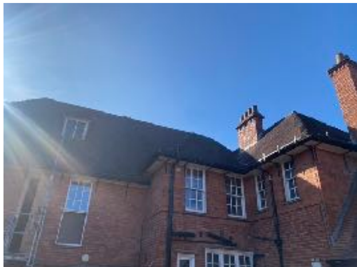
North east elevation of building
