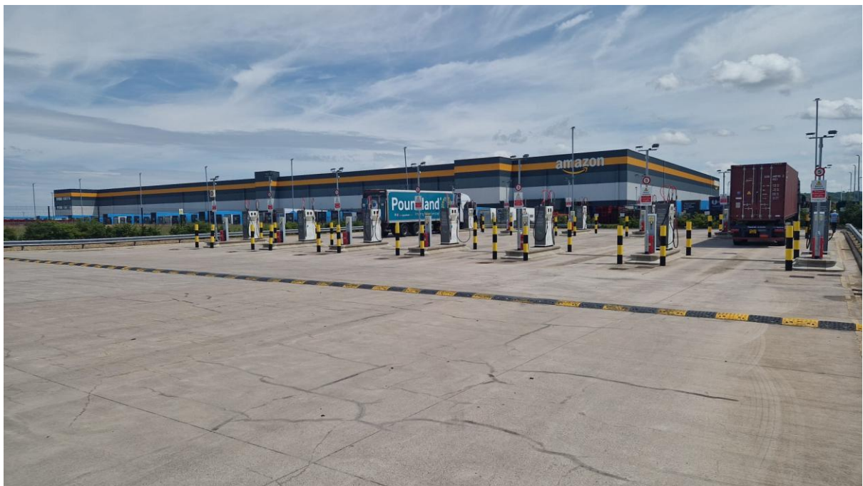
Wide Angle View of Fuel Dispensers
