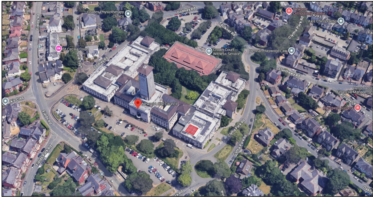
Figure 1 – Google Maps Image. Location of Newport Civic Centre - Glass Rooflight
