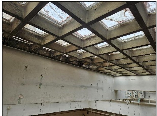
Photograph 4 – Showing section of Glass Rooflight
