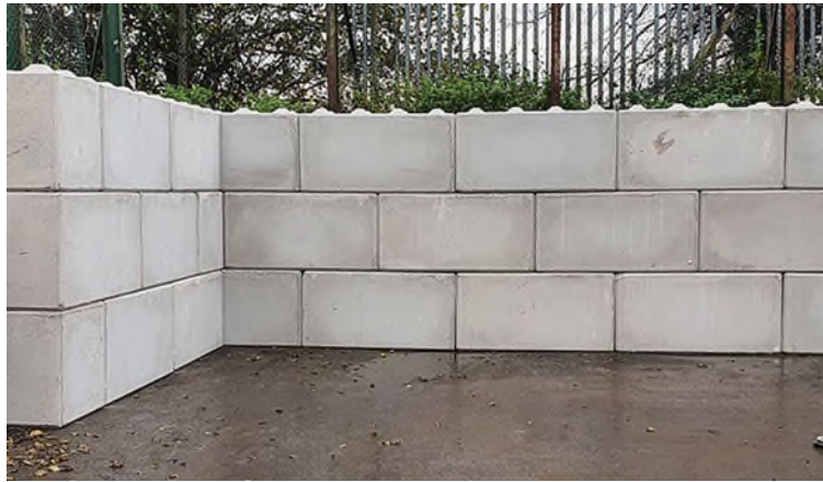
Figure 2 – Legato Block Wall Bay
