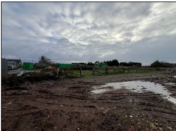
Figure 9: Bare Ground Proposed for Concreting.
