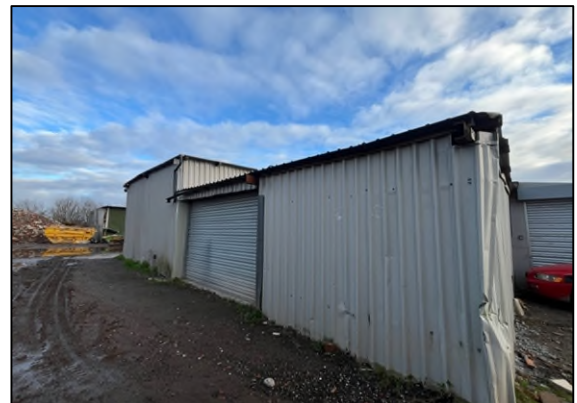
Figure 13: Example of Structures On Site.
