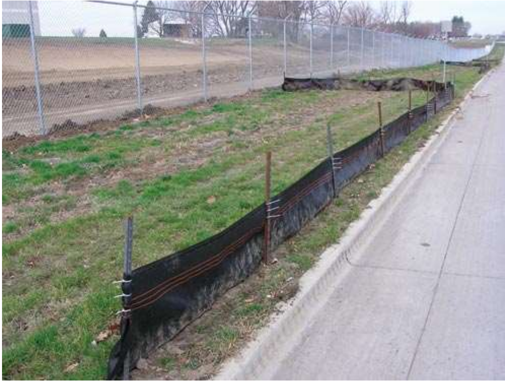
J-hooks create ponding area for sedimentation.
