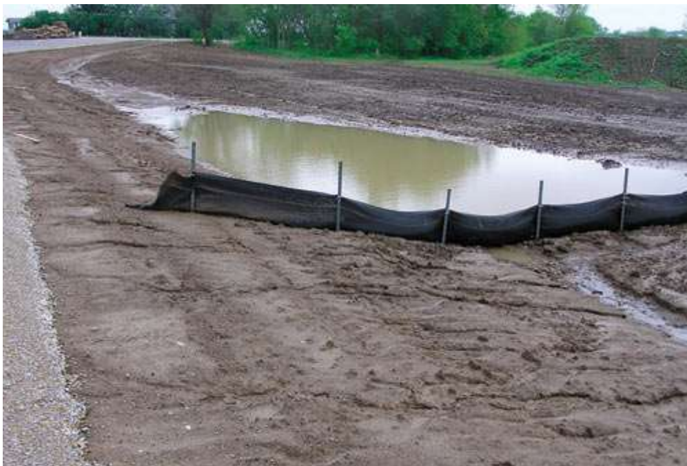
A properly installed silt fence retaining runoff for sedimentation to occur.
