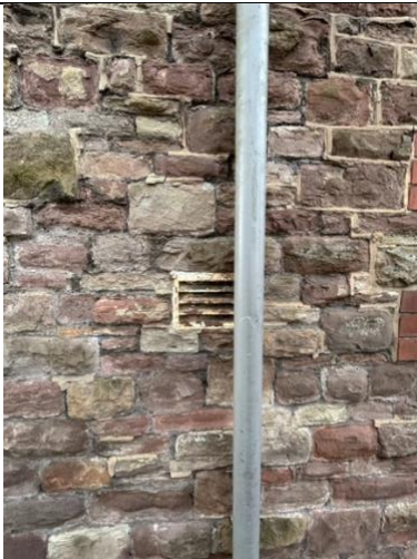
Weathered stone – various mortar type and condition – including cement mortar
