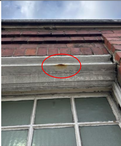
Evidence of spot corrosion to steel beam along edge.
