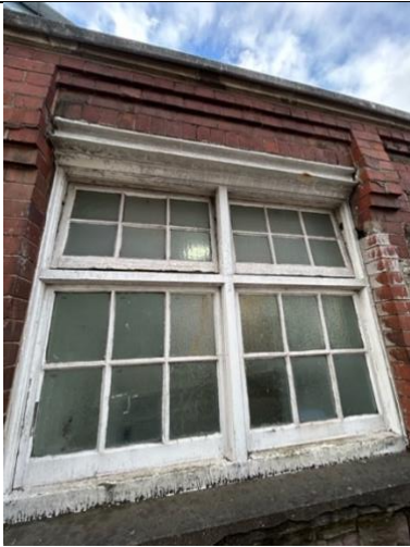
Boys WC window (W2) – timber window with steel lintel above embedded into the wall
