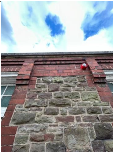
Brick and stonework between windows 1 & 4
