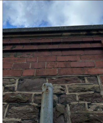
Brick detail above stone – top rows of brick sit below a stone capping – currently dressed in a modern roof finish edge.
