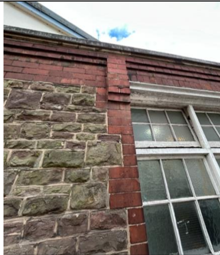
Brick detailing around window
