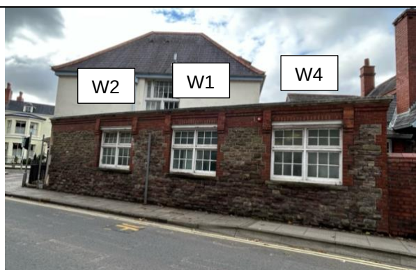
External wall along High street - WCs (Boys & Girls) & entrance lobby windows.
