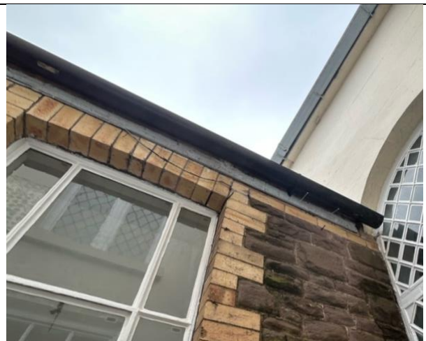
Gutters replaced – temporary provisions
