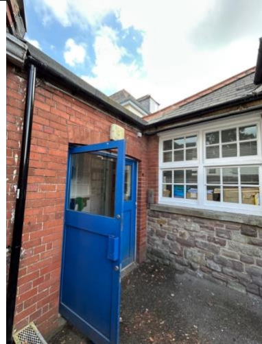
Gutters and downpipe removed – temporary rainwater goods
