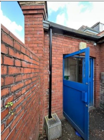
Gutters and downpipe removed – temporary rainwater goods
