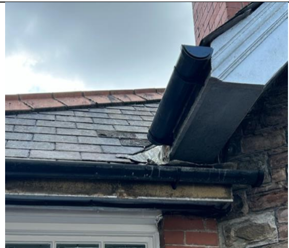
Temporary rainwater goods
