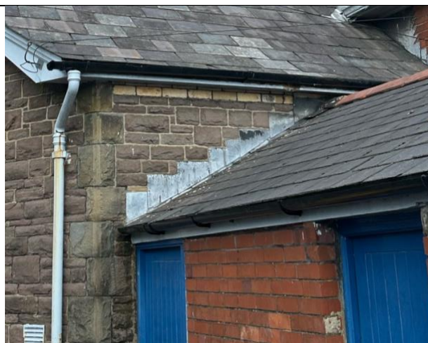
Temporary rainwater goods
