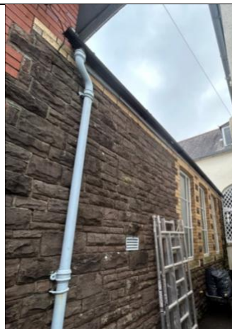
Gutters replaced – temporary provisions – downpipe remains in place will be treated in-situ
