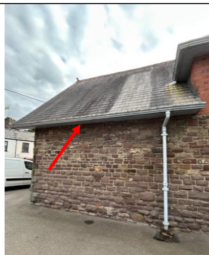
Existing rainwater goods
