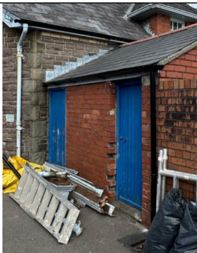
Temporary rainwater goods
