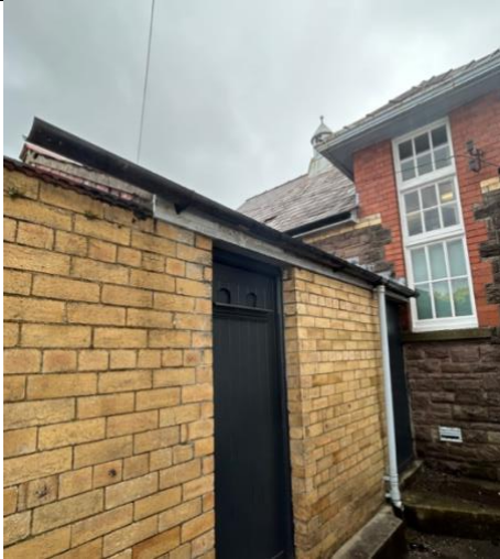
Temporary provisions - gutters
