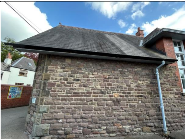
Temporary rainwater goods
