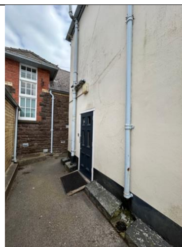
Rainwater goods to rear of school house
