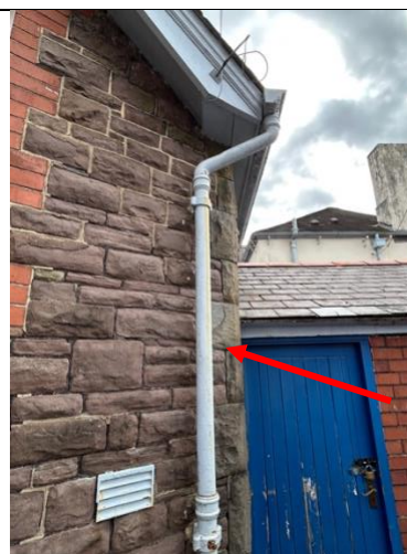
Downpipe off courtyard
