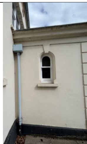
Left side elevation of porch – hopper and downpipe
