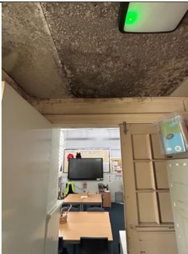
Porch ceiling – previously replaced
