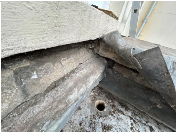
Small drainage outlet through the roof deck / wall. Discharges into a hopper. Potentially blocked / damaged within the structure
