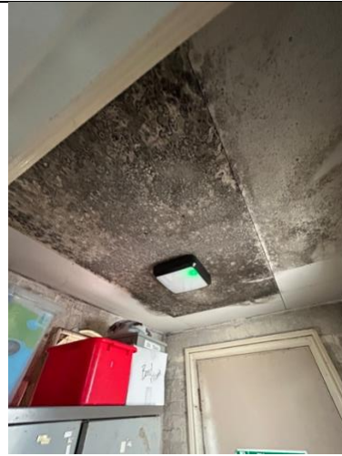
Porch ceiling – previously replaced
