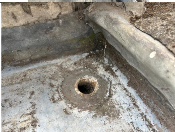
Small drainage outlet
