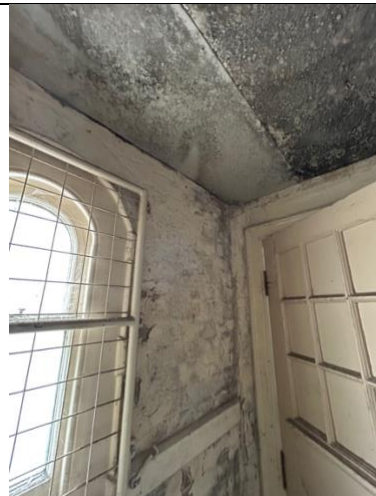
Porch ceiling – previously replaced
