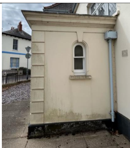
Right side elevation of porch – hopper and downpipe
