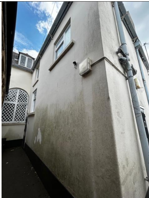
Rear elevation – Access to stairwell
