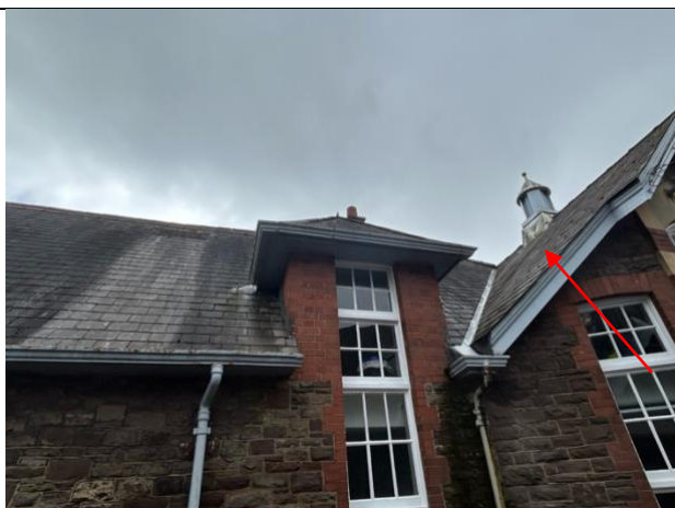
Roof area over courtyard to be assessed during summer work – gable left slope
