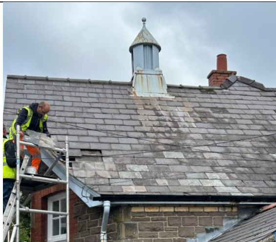
Emergency slate repairs over Easter 2025 – Salvaged Welsh slate provided
