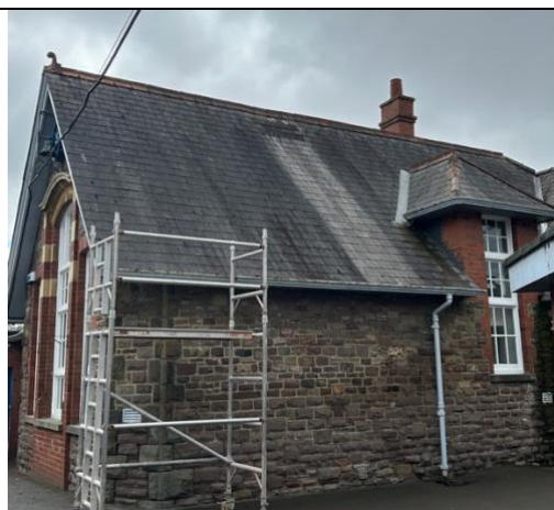
Roof area over courtyard to be assessed during summer work
