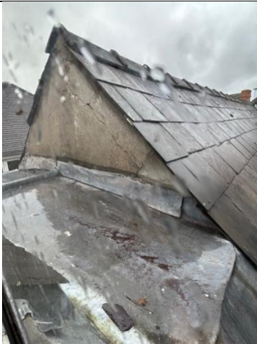
Lead roof to be reviewed – render replaced
