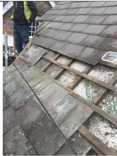
Emergency repairs undertaken over Easter – Some areas of Kingspan insulation previously provided
