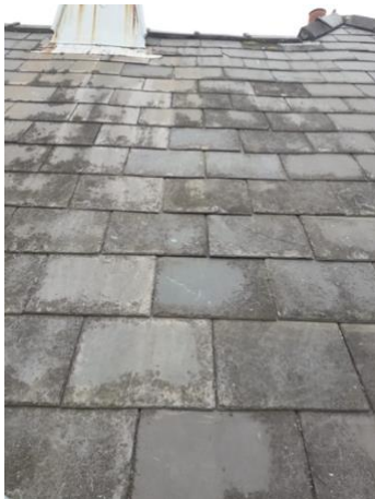
Emergency repairs undertaken over Easter
