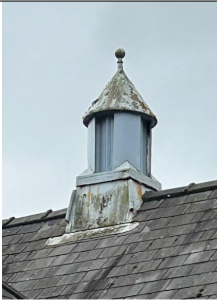
Ventilation dome to be removed temporarily for repair and assessment. To be reinstated as a feature. Left slope
