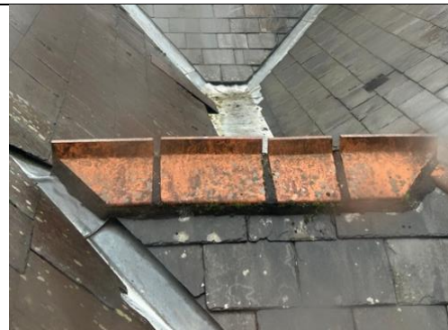
Ridge to rear dormer – Clay plain crested flat top ridge
