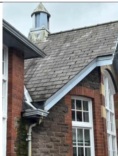
Courtyard gable roof left slope – to be replaced over summer
