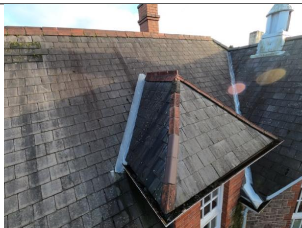
Dormer roof to front courtyard to be reviewed during summer work
