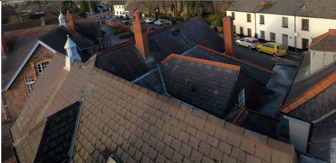
Rear roof areas – to be assessed once scaffold is in place
