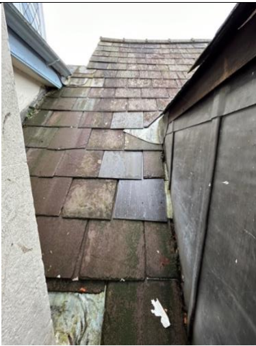
Replace slates to back slope with new Glendine
