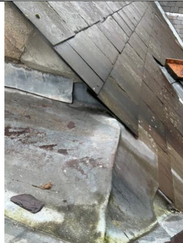
Review lead detail at roof line
