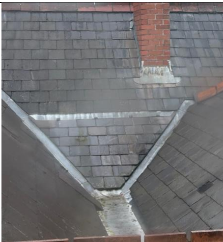
Assess lead valleys – Allow for replacement
