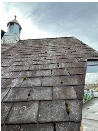
Courtyard gable roof left slope
