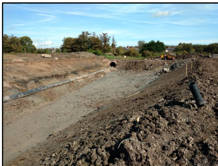
Figure 1: Preparation works for lining of the reën.
