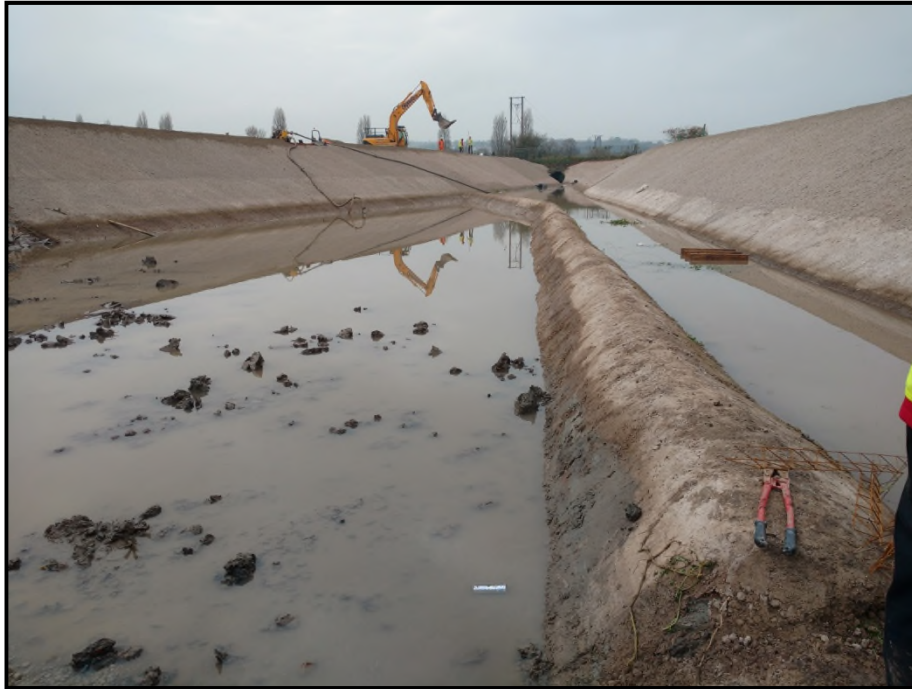
Figure 2: Newly lined reen (03.11.2017)
