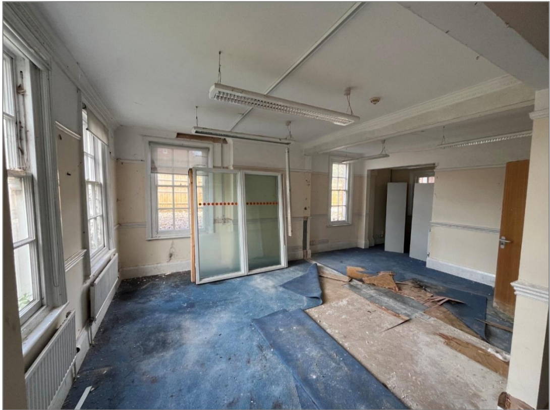
Photo 25: View northwest into the main front room on the northwest side of the main house.
