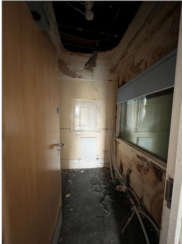
Photo 28: View northwest into small side room from corridor.
