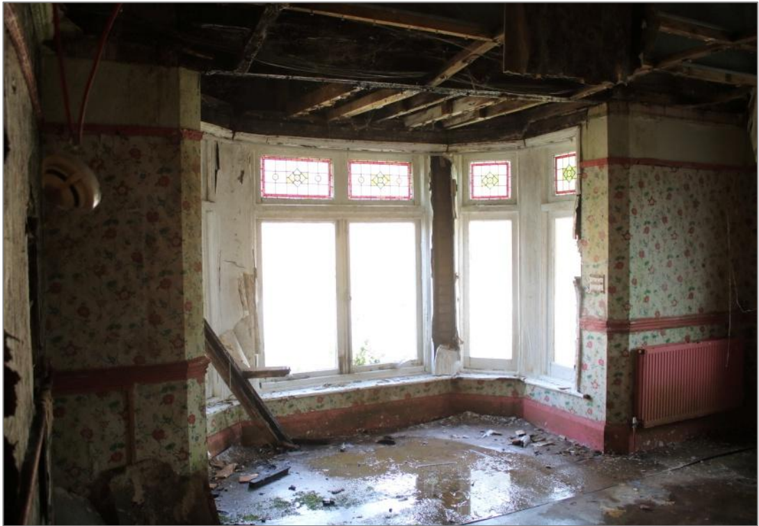
Photo 43: View northwest of the bay window in the single-storey extension.
