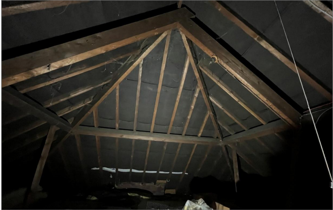
Photo 57: View northwest of the roof structure.
