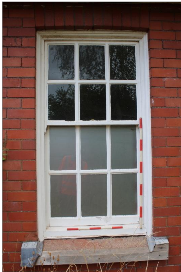
Photo 4: View northeast, detail of ground floor sash window. 1m & 0.5m scale.
