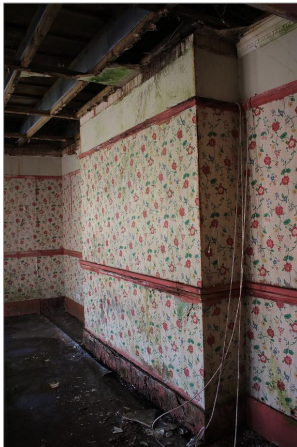
Photo 44: View east of the former fireplace in the single storey extension.
