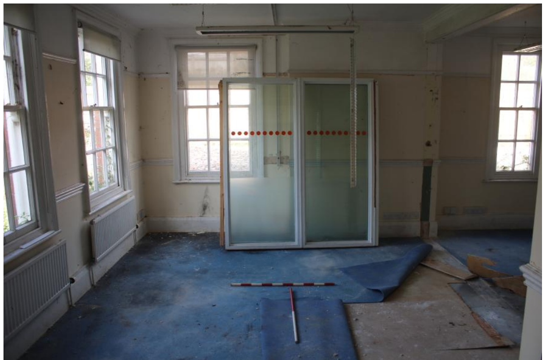
Photo 26: View northwest of main front room to the northwest. 1m scales.
