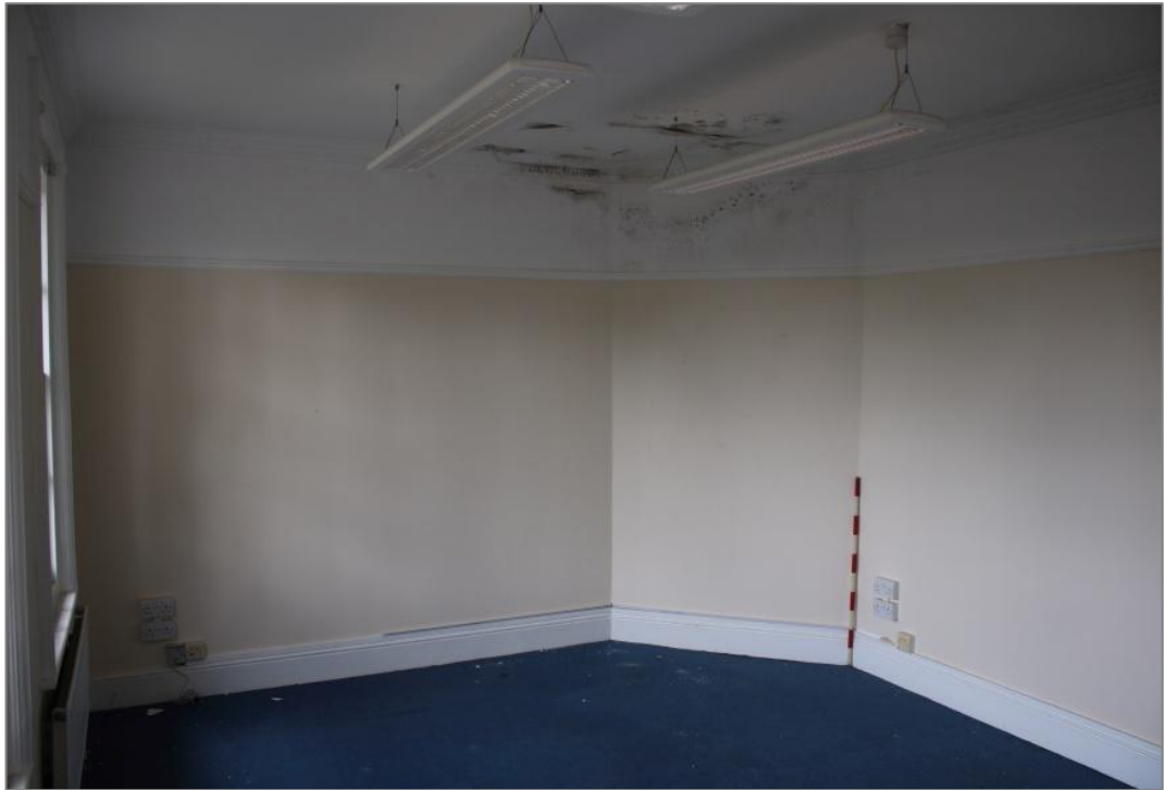
Photo 50: View northwest of blocked corner fireplace in Bedroom 2. 1m scale.
