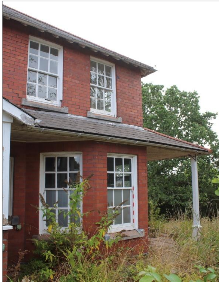
Photo 5: View east of ground floor bay window. 1m scale.
