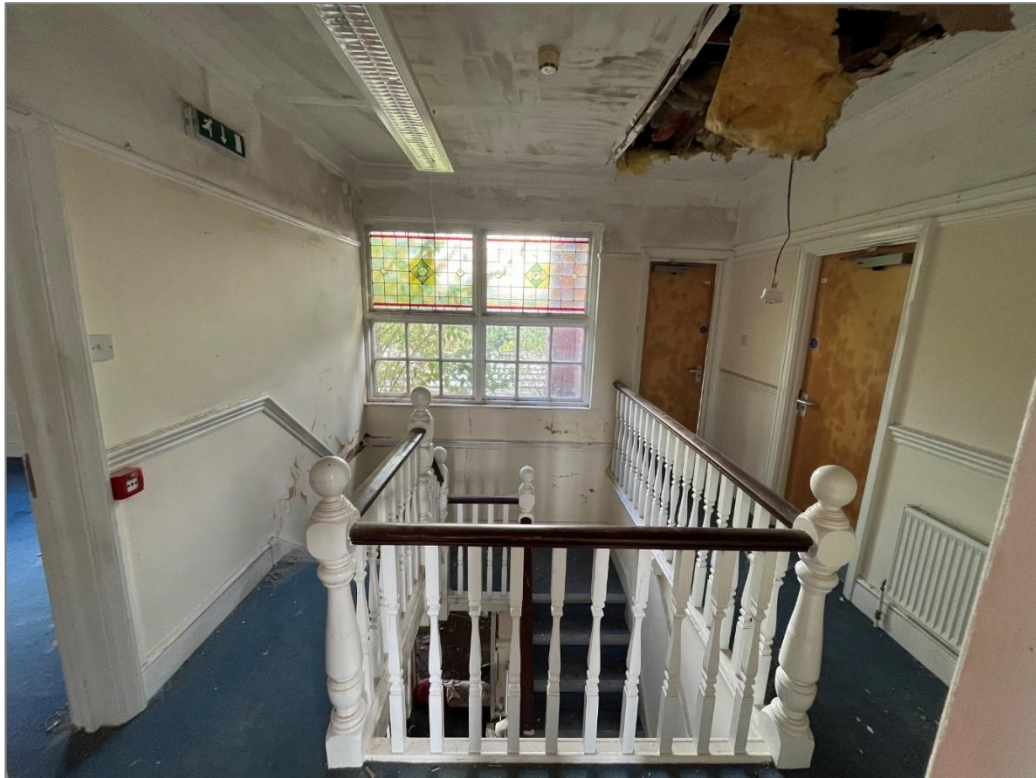
Photo 46: View northeast of the 1st floor landing.
