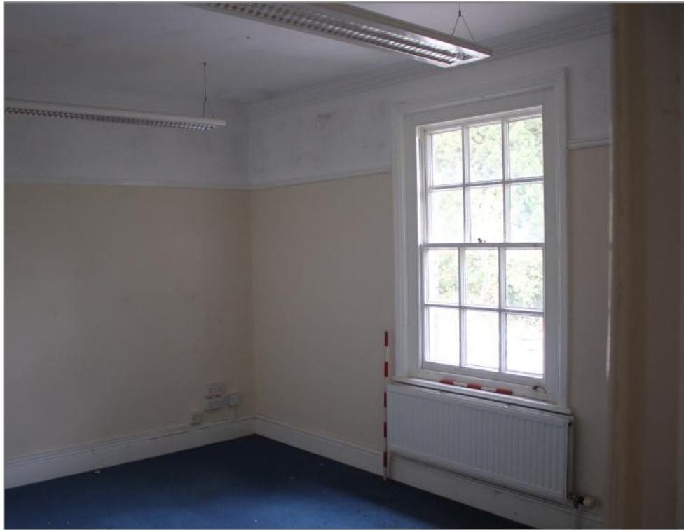
Photo 48: View north of detail within Bedroom 1. 1m & 0.5m scale.
