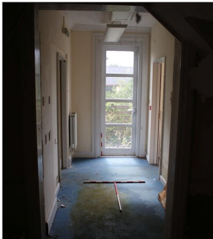
Photo 34: View southeast of rear corridor. 1m & 0.5m scale.
