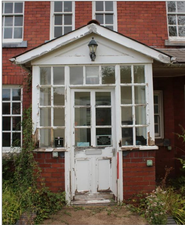
Photo 3: View northeast, detail of the entrance porch. 1m scale.
