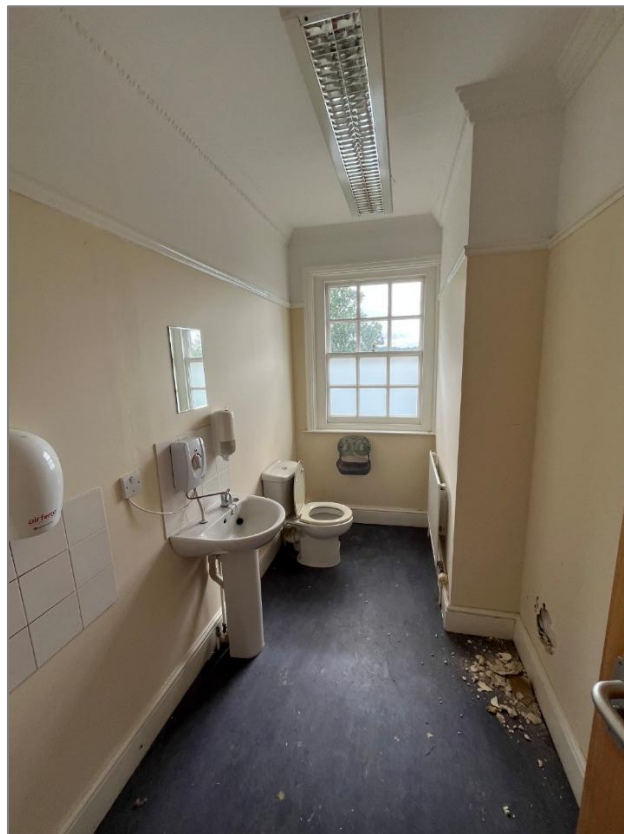
Photo 53: View southeast of the 1st floor toilet.
