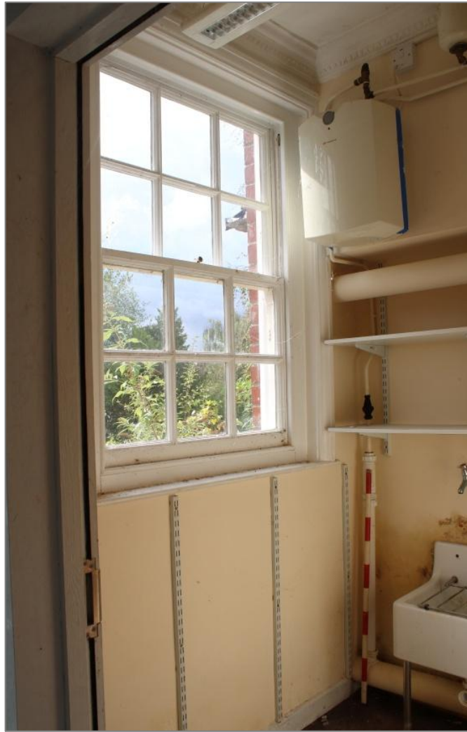
Photo 36: View south into the small rear room. 1m scale.
