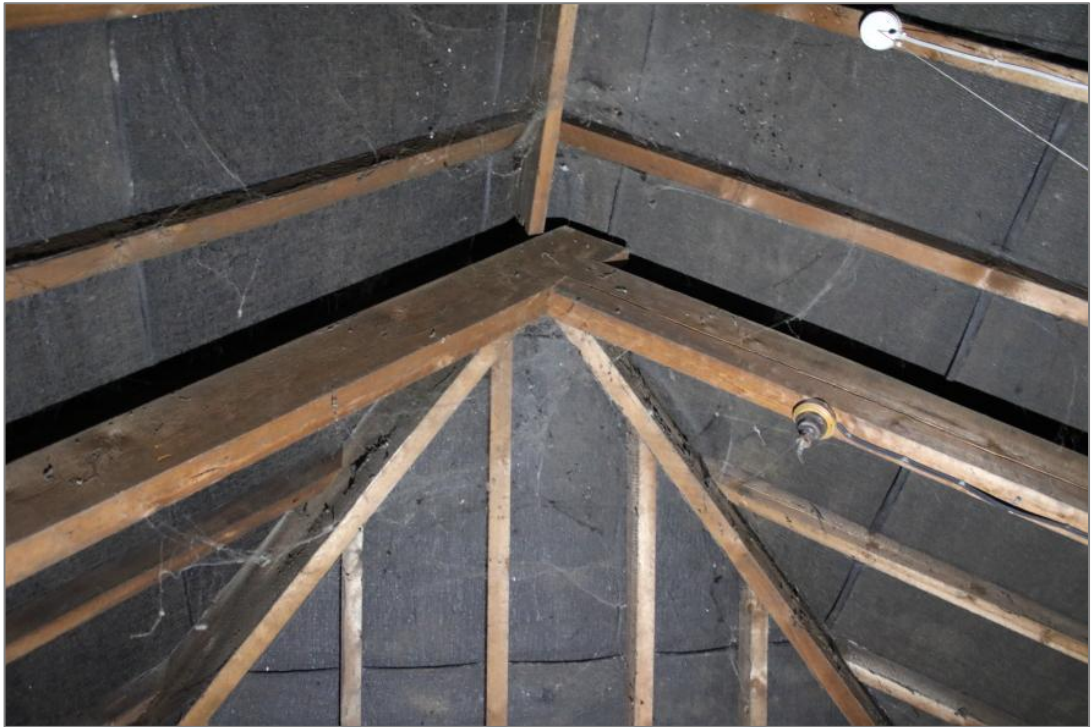
Photo 59: Detail of roof structure joints.
