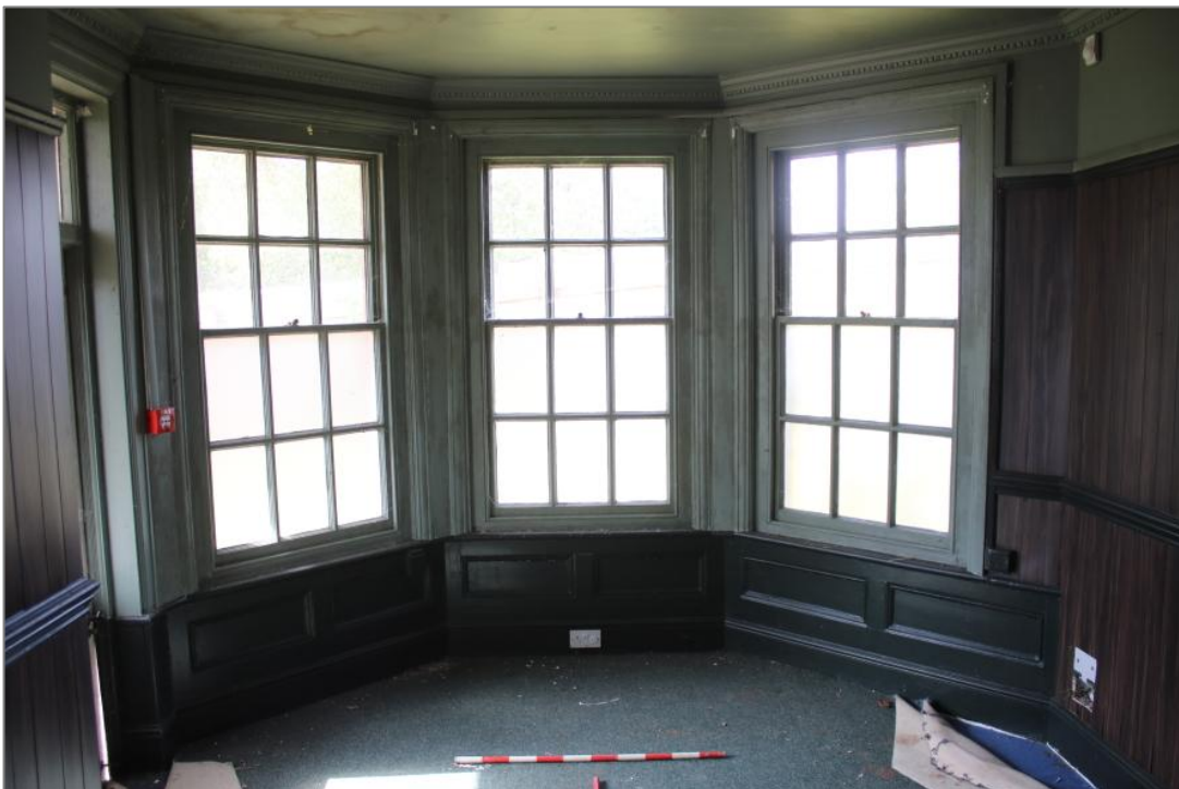
Photo 32: View southwest of the internal side of the bay window. 1m scale.
