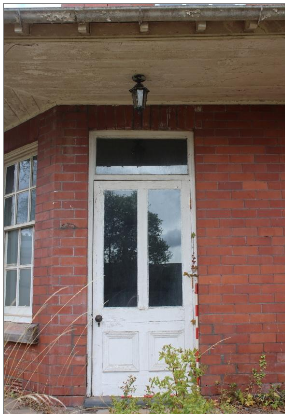
Photo 8: View northeast showing the doorway from the bay-fronted room. 1m & 0.5m scale.
