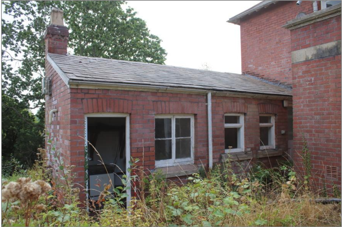
Photo 17: View southeast of the service range extension to the rear of Felthorpe House. 1m scale.
