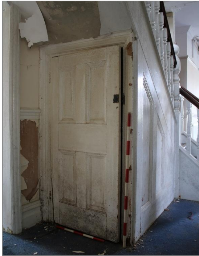
Photo 24: View southwest, understairs cupboard. 1m & 0.5m scale.
