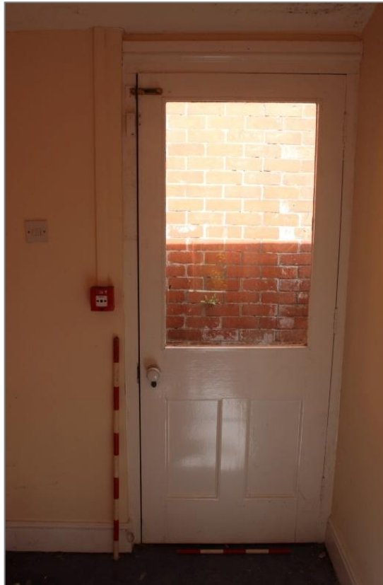
Photo 40: View northwest of opposing door in rear service wing corridor. 1m & 0.5m scale.
