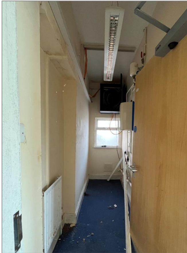
Photo 37: View northeast into narrow room on northeast side of corridor.
