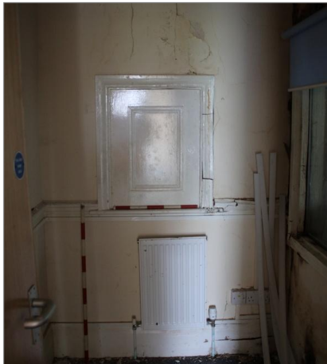
Photo 29: View northwest, detail of former serving hatch in small side room. 1m & 0.5m scale.
