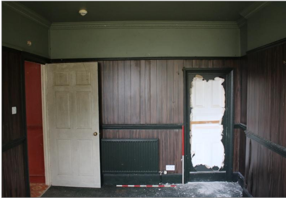
Photo 33: View northeast of the blocked doorway in the front bay window room. 1m scales.
