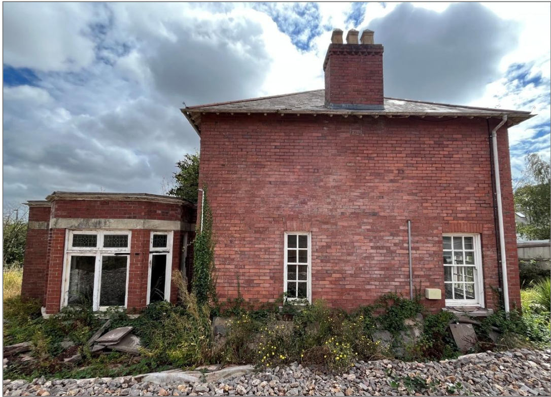
Photo 12: View southeast of Felthorpe House.
