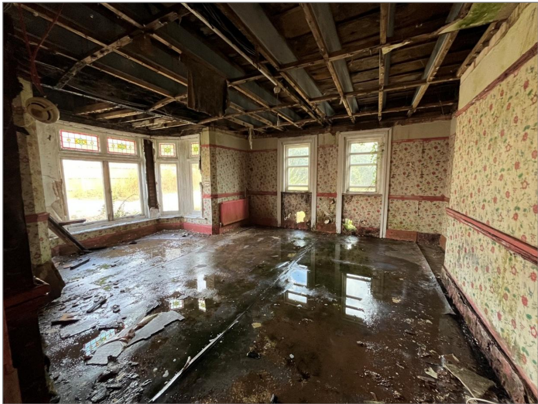
Photo 42: View northeast into the room occupying the single-storey extension.
