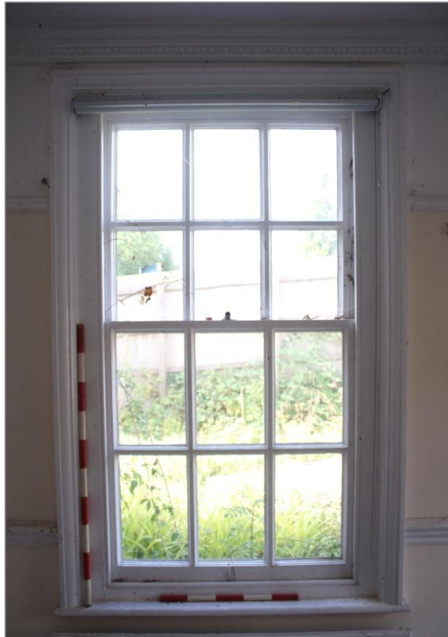
Photo 27: Detail of internal face of sash window in the front wall. 1m & 0.5m scale.
