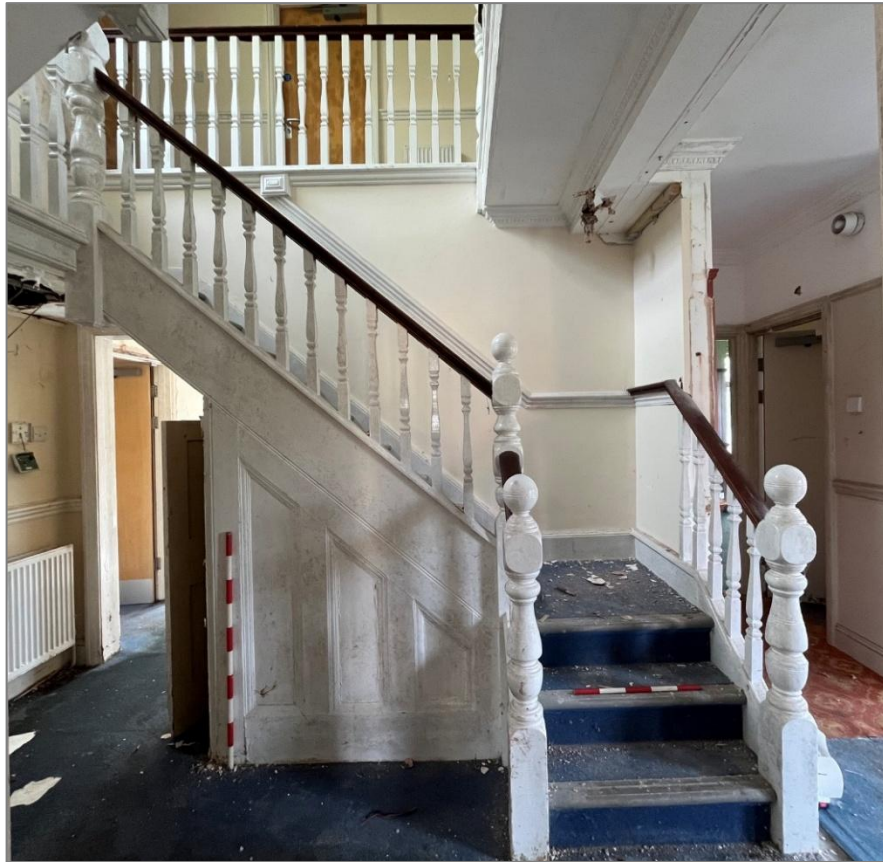
Photo 22: View southeast of the stairway at ground floor level. 1m & 0.5m scale.
