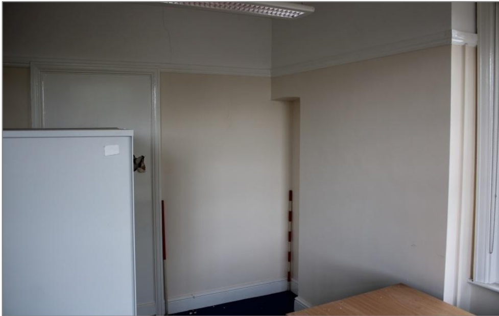
Photo 52: View northeast in Bedroom 3, showing the block fireplace on the right, and blocked door on the left, all obscured by modern office furniture. 1m scales.
