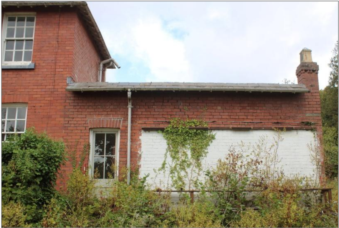
Photo 11: View northwest, detail of the later service range extension.
