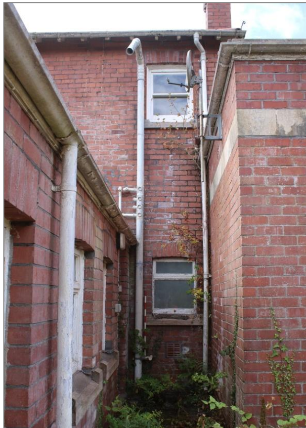
Photo 16; View southwest of the original house visible between the two later extensions. 1m scale.
