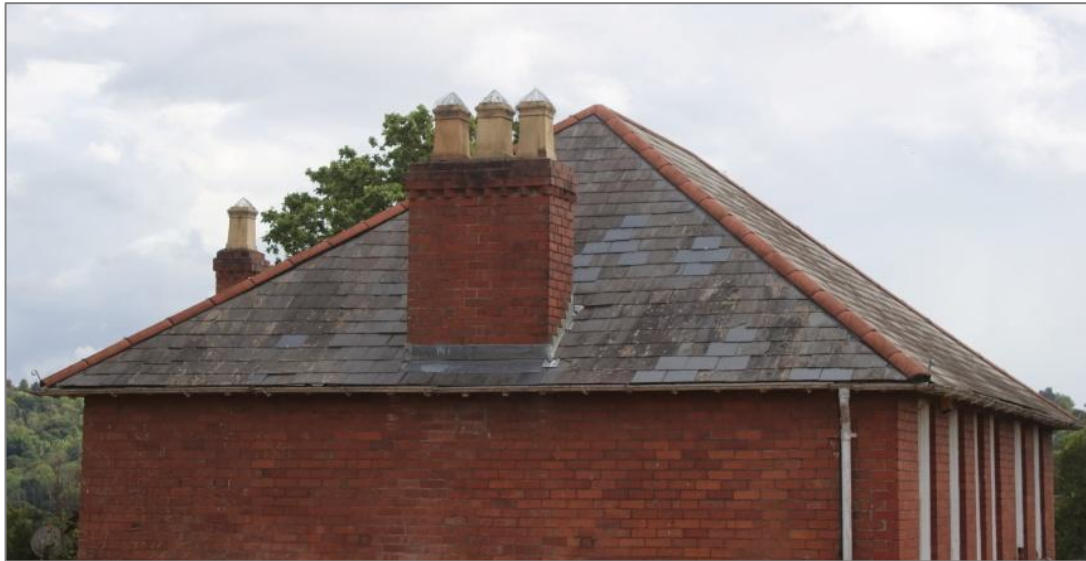
Photo 14: View southeast showing detail of the chimney stack on the northwest face.
