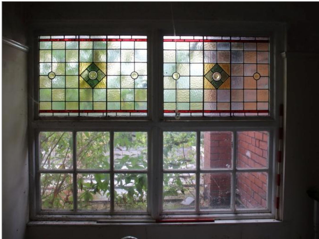
Photo 45: View northeast of the stairwell window. 1m scales.
