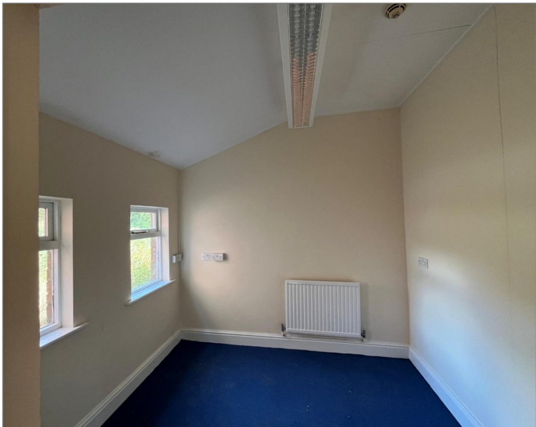
Photo 41: View northeast into rear service wing room.
