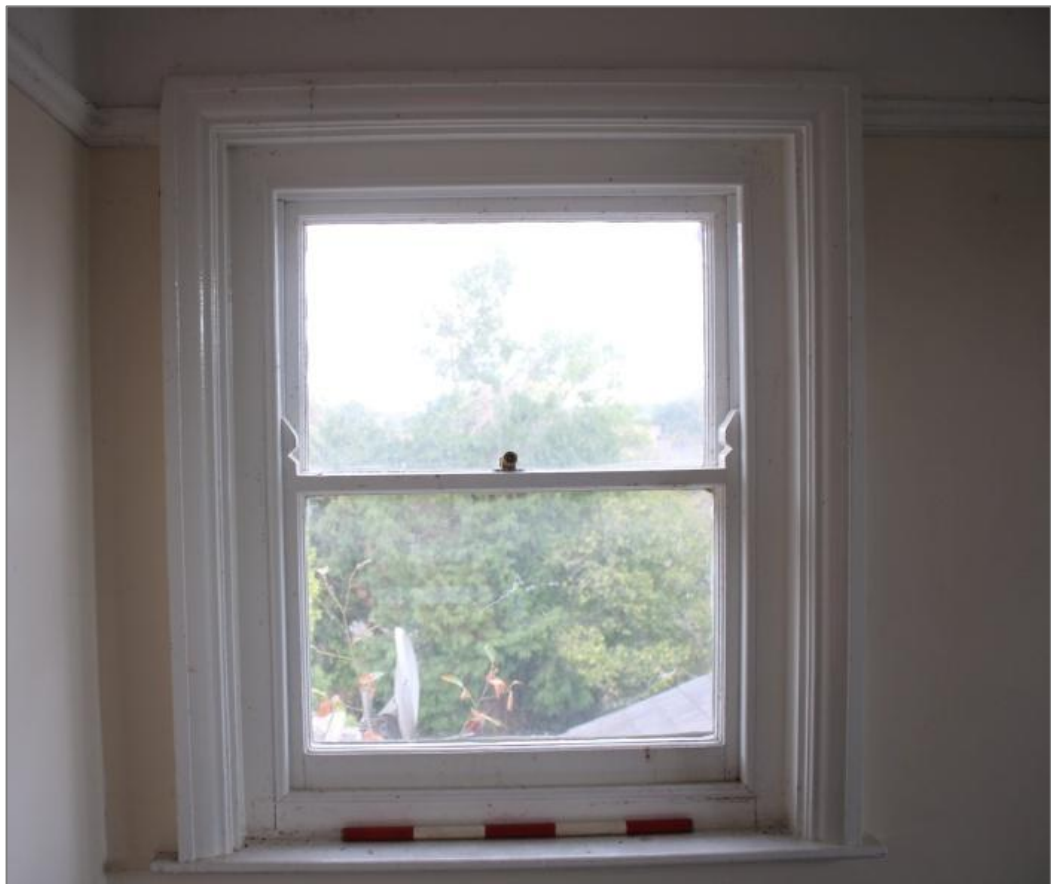
Photo 56: View northeast, showing window detail in Bedroom 5. 0.5m scale.
