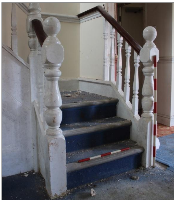
Photo 23: Detail of stair newel and balusters. 1m & 0.5m scale.
