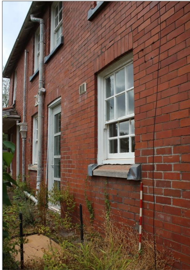
Photo 9: View west along the garden face of the house, showing the reduced height sash window. 1m scale.
