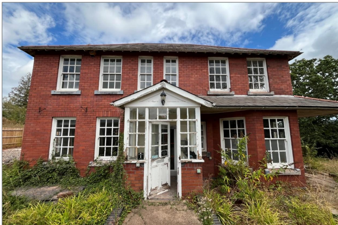
Photo 2: View northeast of the front face of Felthorpe House.
