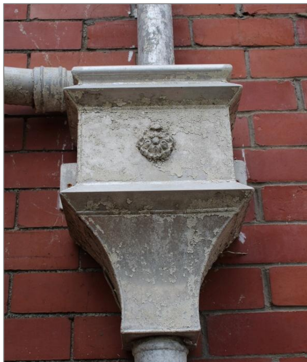
Photo 10: Detail of the rainwater hopper on the garden face of the house.
