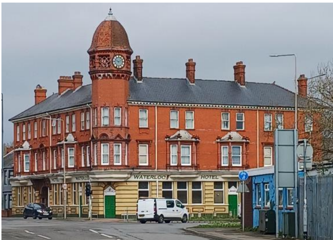
Illus 7. Waterloo Hotel Grade II Listed (18182) within Waterloo Conservation area, looking north from port entrance.
