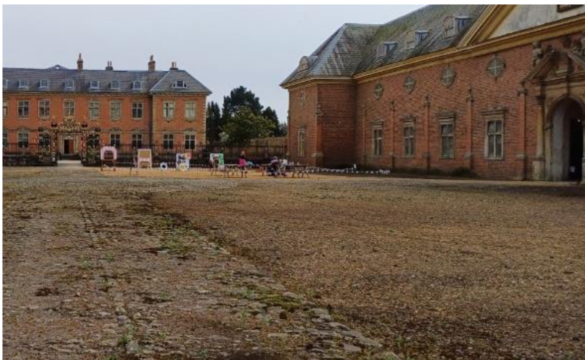
Illus 16. Tredegar House Grade I Listed Building (2902) left, Stable Block and Orangery Grade I Listed (2910) right, looking south-east
