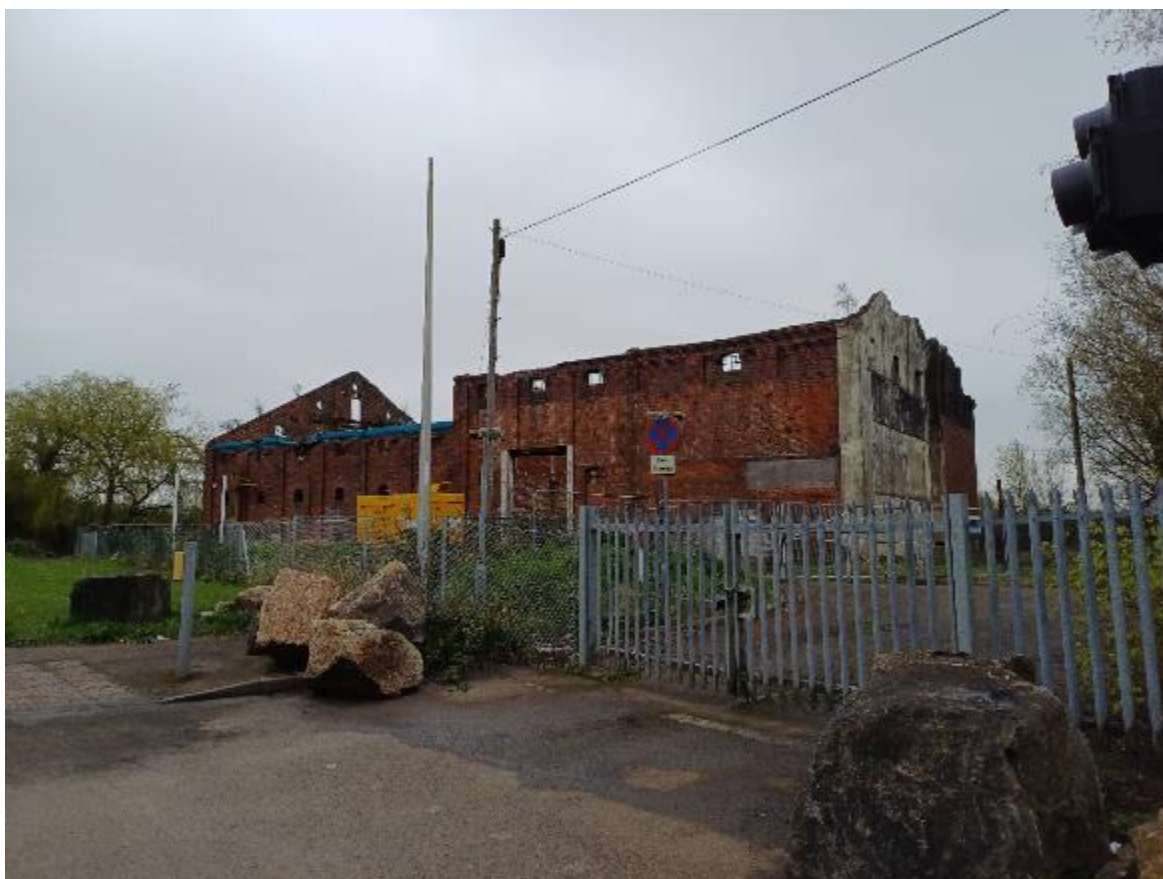
Illus 12. Malt House Grade II Listed (18178), looking south-east.
