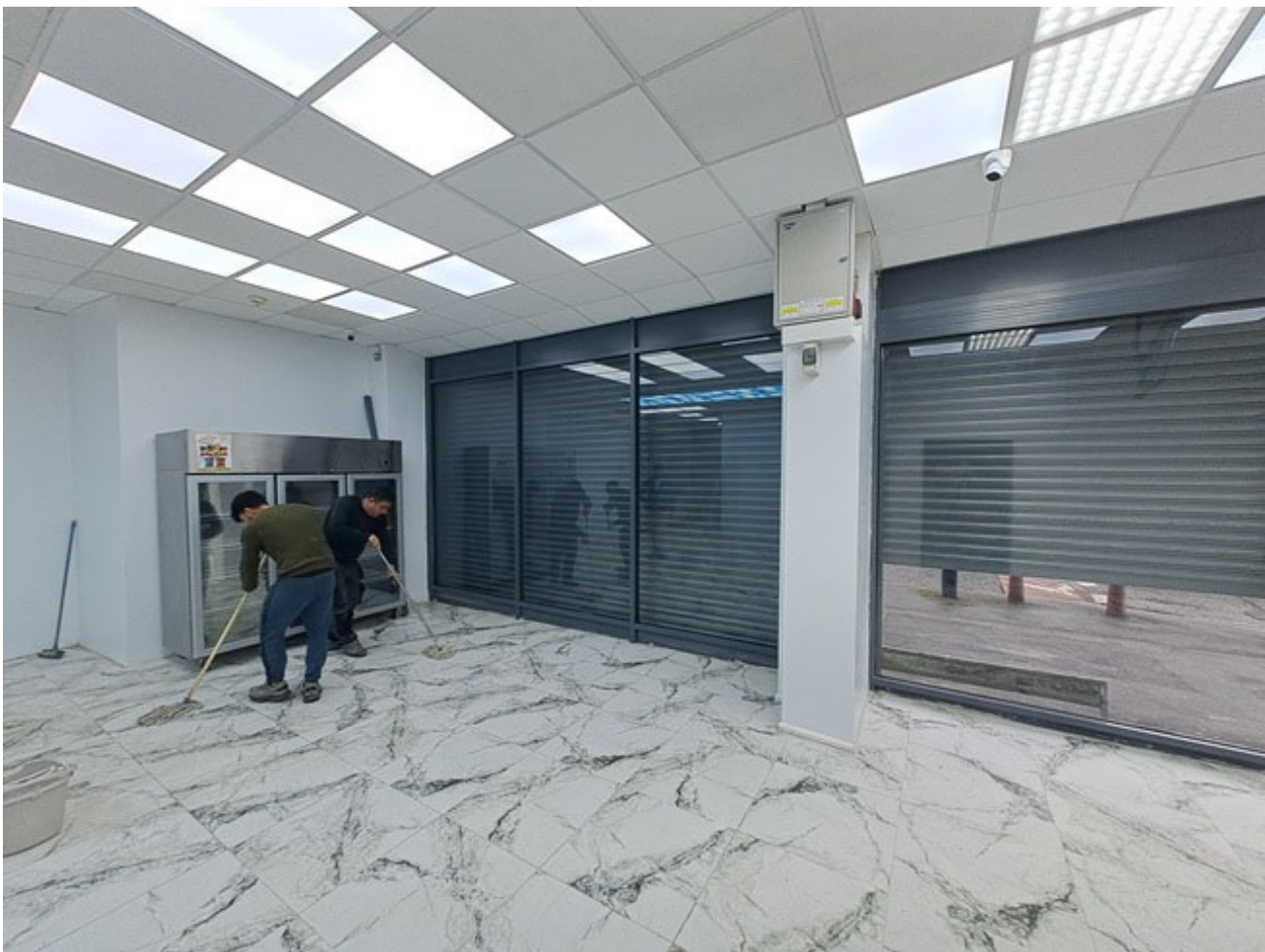
Photo 4 – New Flooring and shop front
