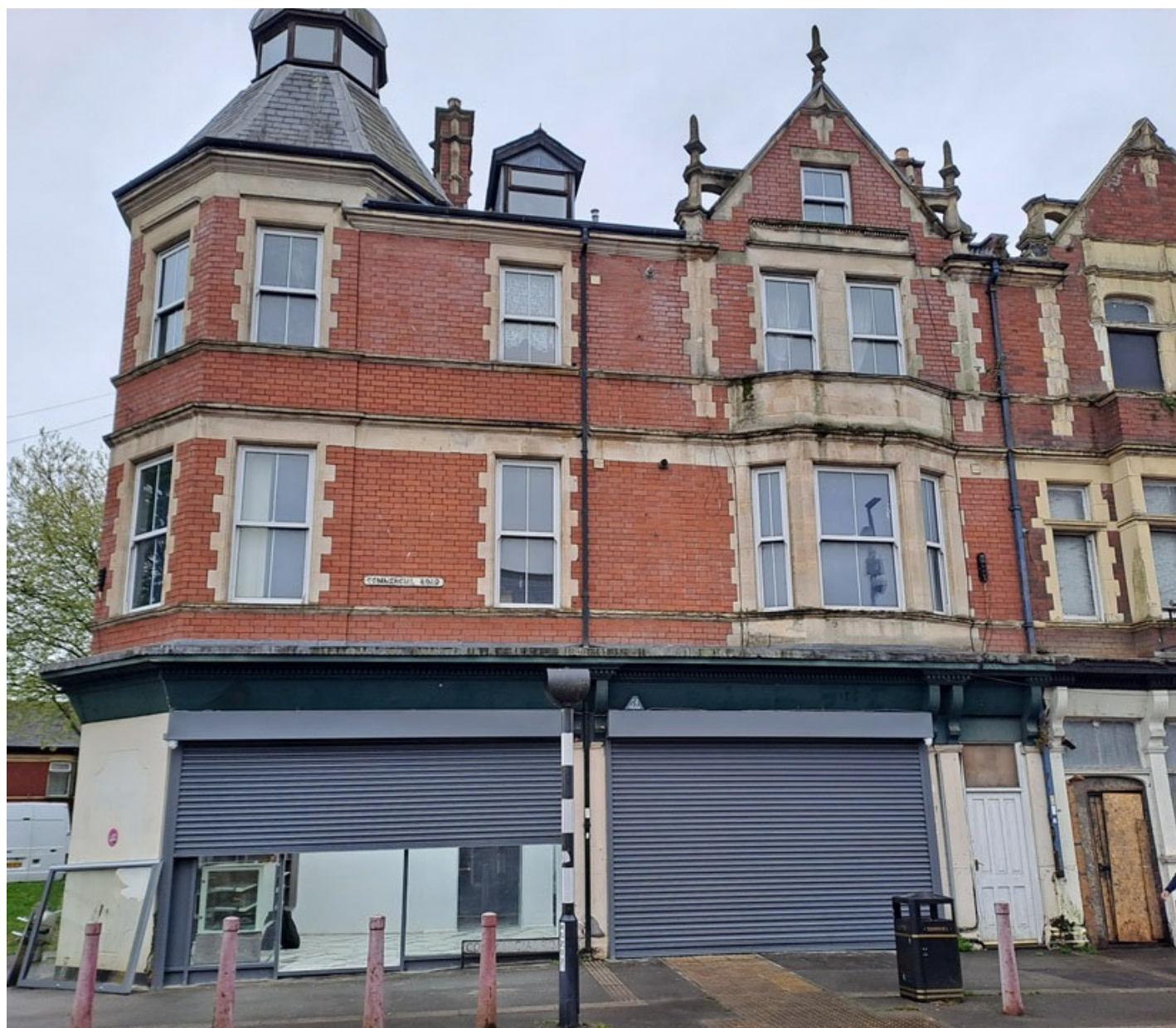
Photo 1 – Front of property
