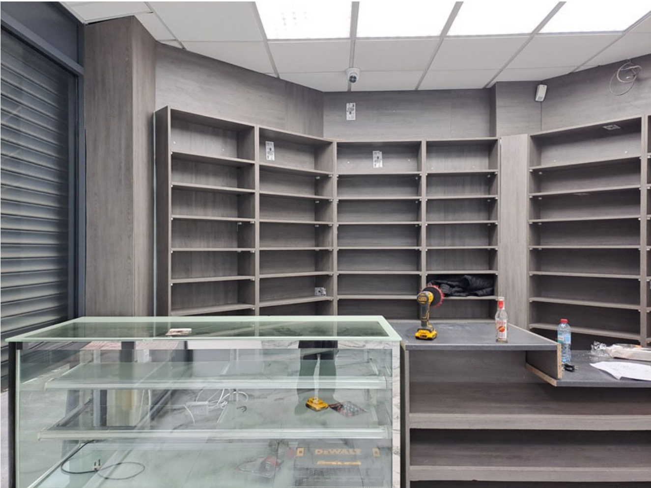
Photo 3 – Shop Fit out
