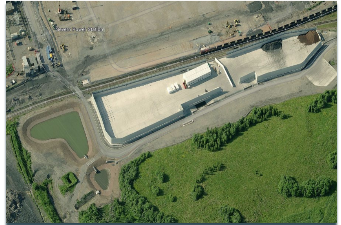
Aerial Image of the Former Uskmouth Power Station
