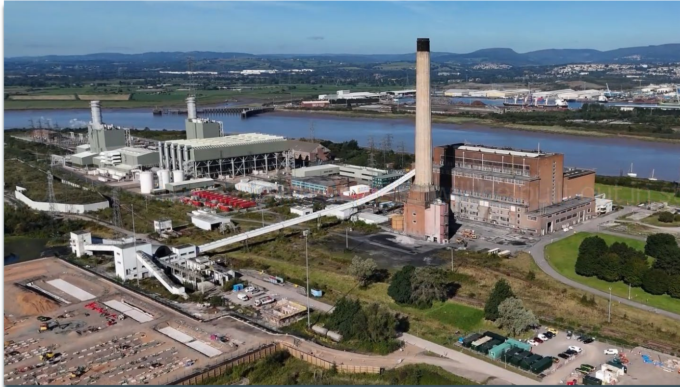
Aerial Image of the Former Uskmouth Power Station
