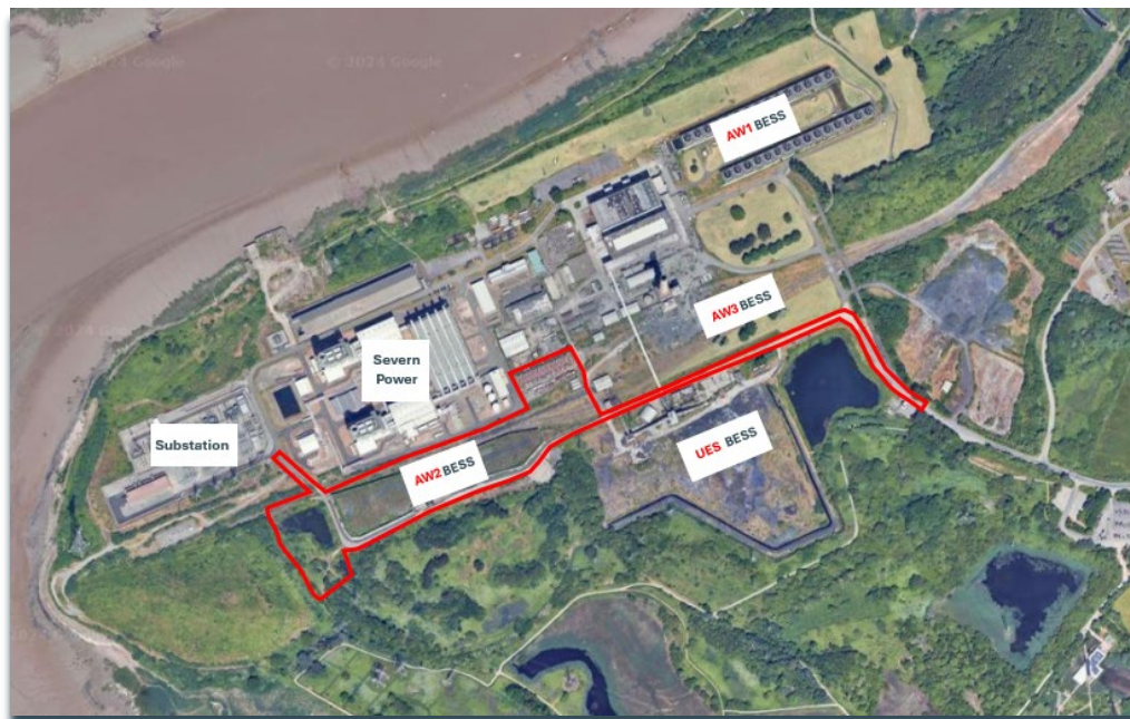
Figure 2: Aerial Image of Proposed BESS Site
