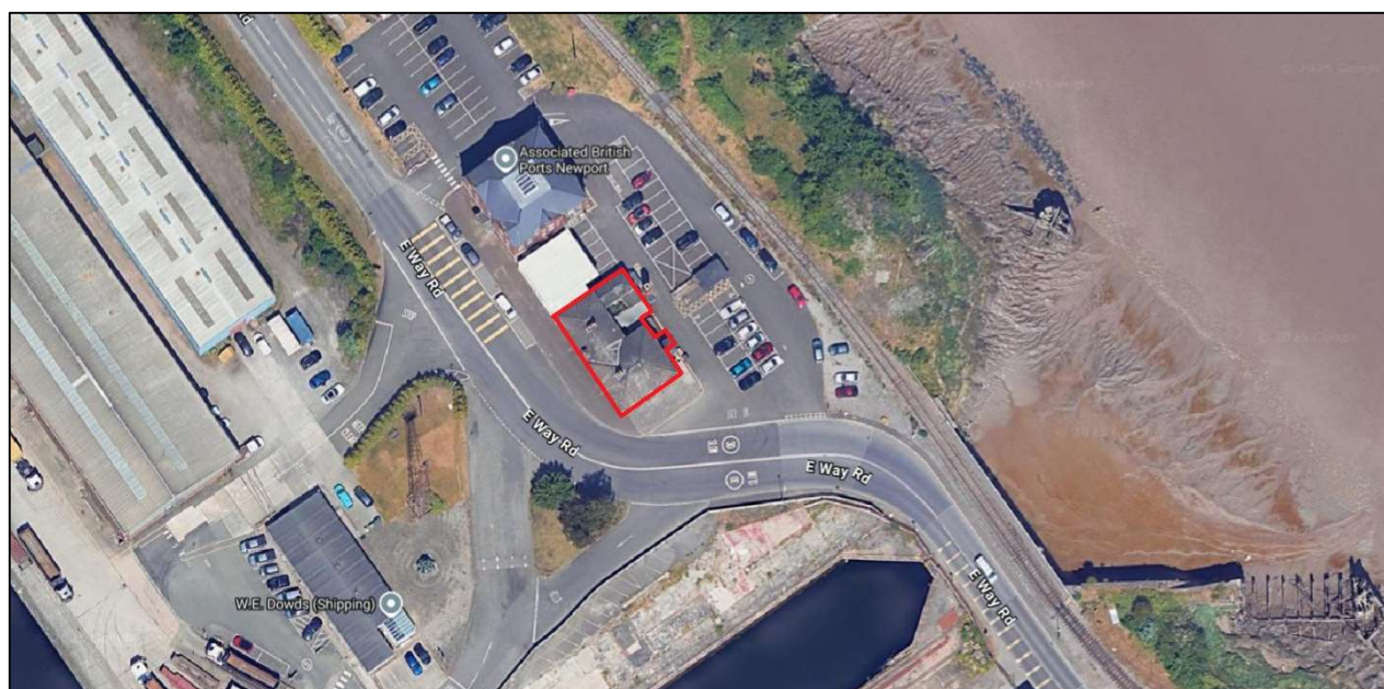
Figure 1 – Survey Building Location (Port Office)
