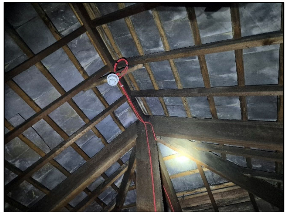
Figure 22 – Underside Roof Detail of (S) Section of Main Loft. The Roof Tiles in this Location have been Set Directly onto Timber Battens, with No Felt Underlay Present
