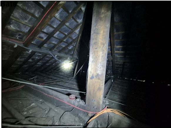
Figure 15 – Gap Around (W) Side of Chimney Breast Enables Access to (S) Section of Main Survey Building Loft
