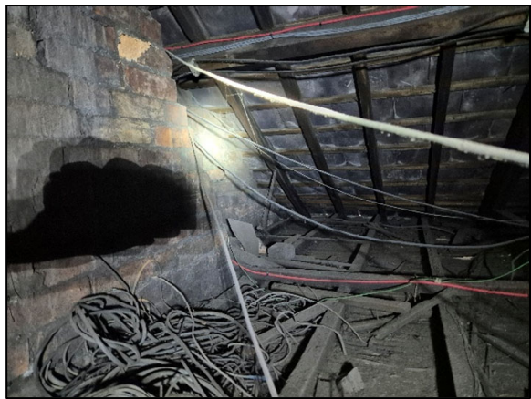
Figure 15 – Gap Around (W) Side of Chimney Breast Enables Access to (S) Section of Main Survey Building Loft
