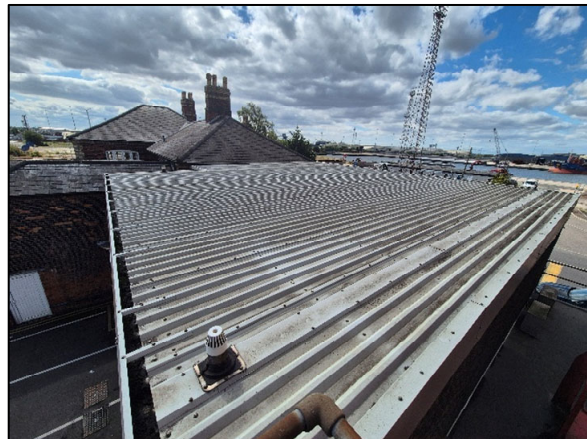
Figure 10 – Roof of Flat Roofed Extension
