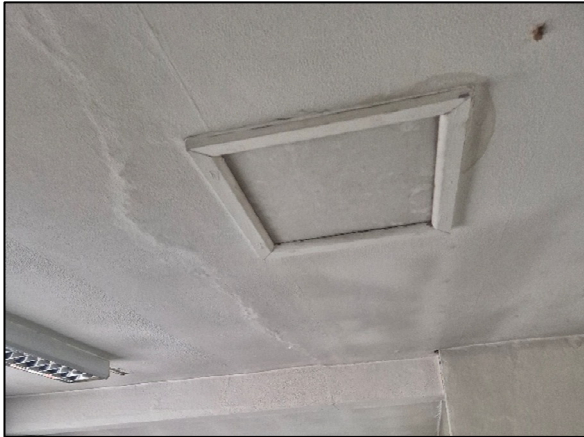
Figure 23 – Access Point to Standalone Small Loft at (NE) of Building
