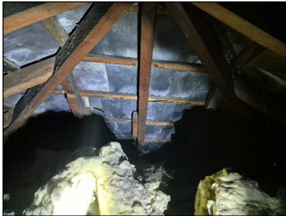
Figure 25 – (NE) Standalone Loft Interior, Looking (NE)
