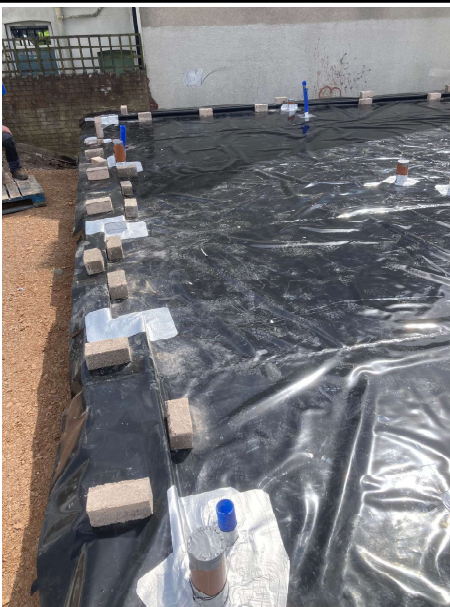
The RTEC 4 Gas Membrane taken over the perimeter block work.
