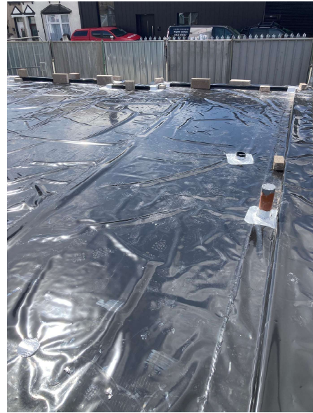
An overview of the installation.
