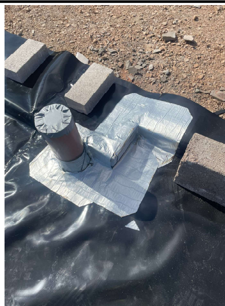
A sealed corner and pipe penetration.
