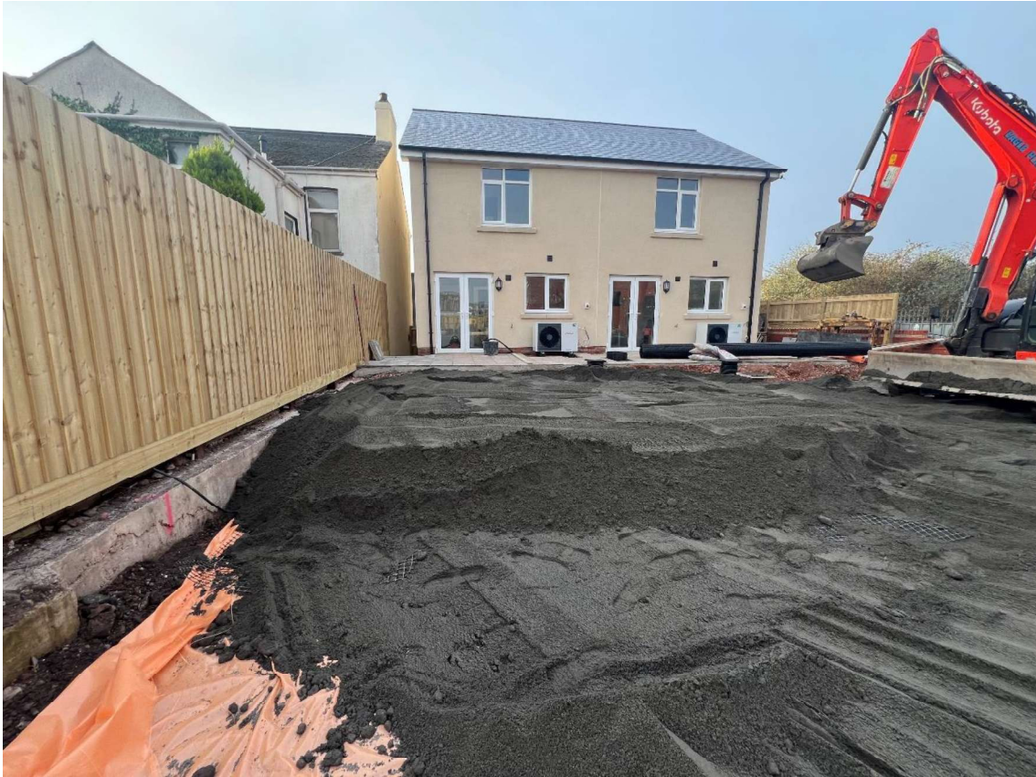
Rear Plot 9 (Left) and Plot 8 (Right) – Membrane & No Dig Mesh with Top Soil
