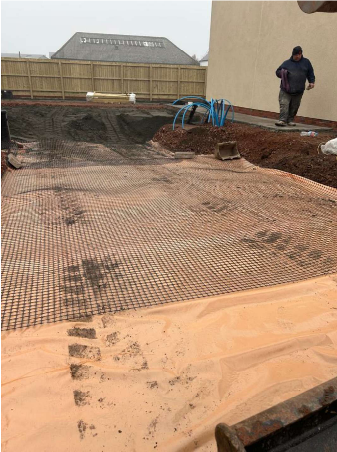
Plot 3 and Plot 4 – Membrane & No Dig Mesh looking towards Plots 5 to 7
