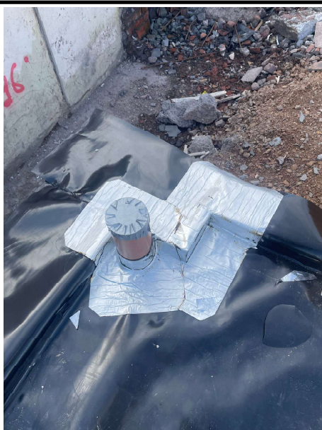
A sealed corner and pipe penetration.
