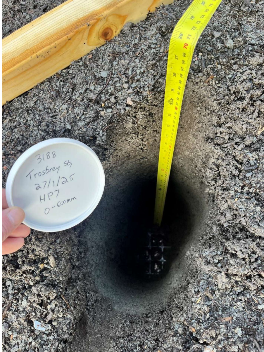
Hand pit excavated in the rear garden of Plot 7.
