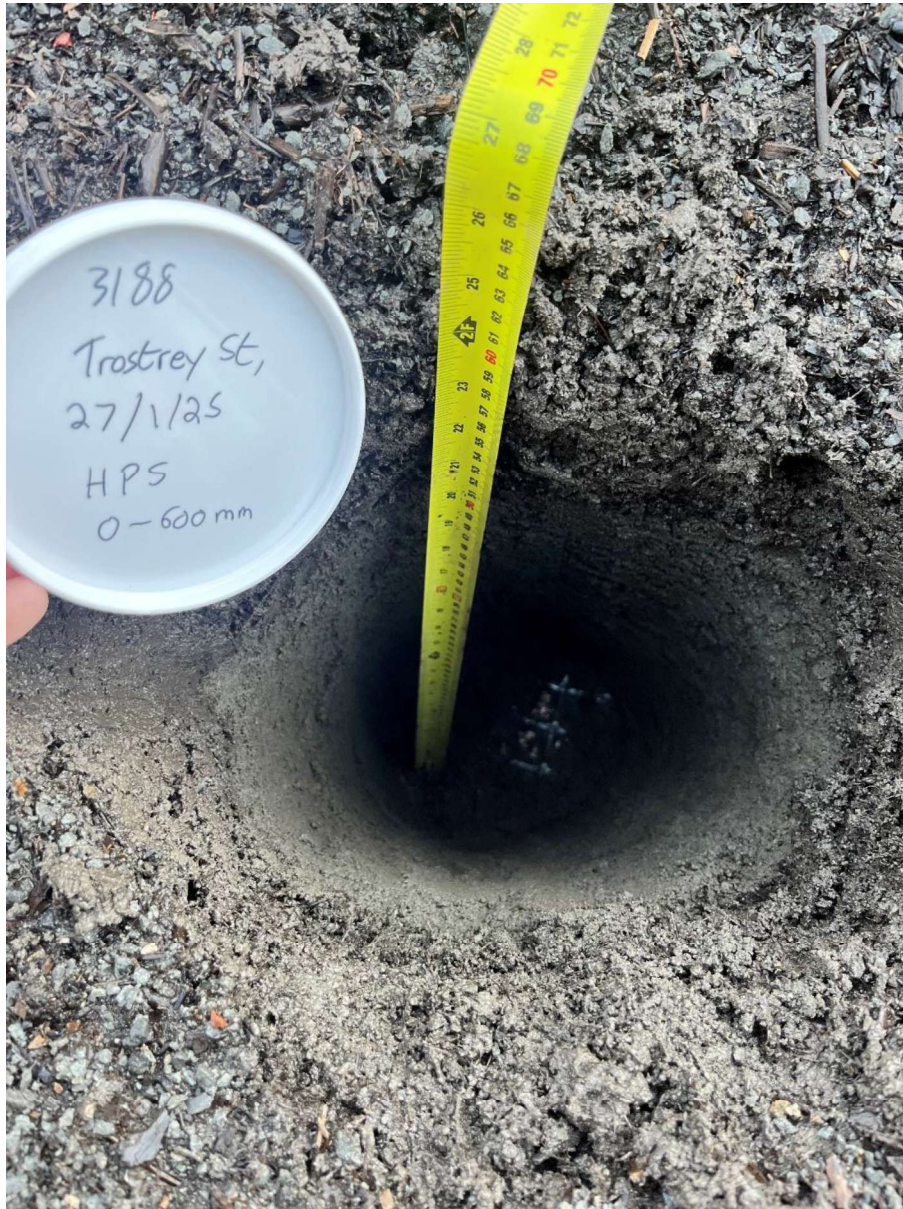
Hand pit excavated in the rear garden of Plot 5.
