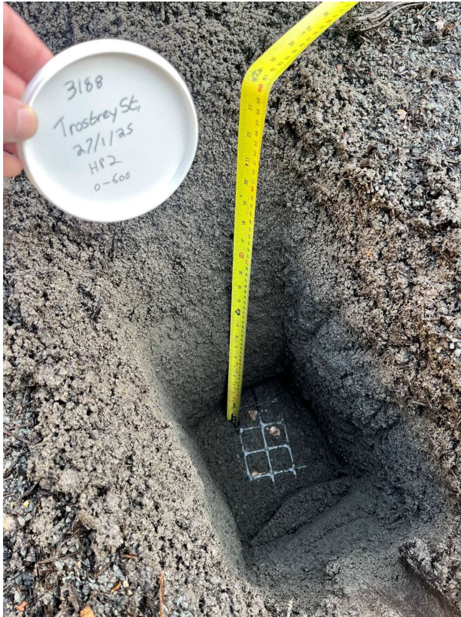
Hand pit excavated in the rear garden of Plot 2.
