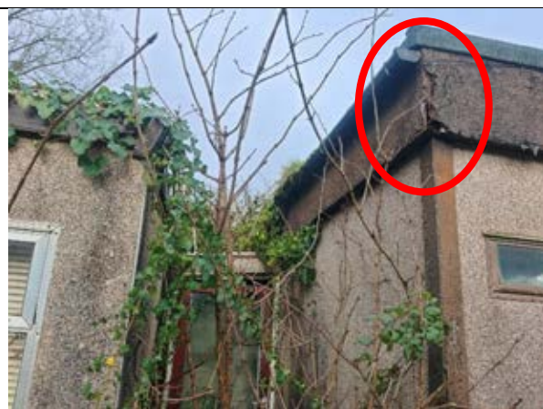
Photo 22: Internal view of B3 showing exposed insulation
