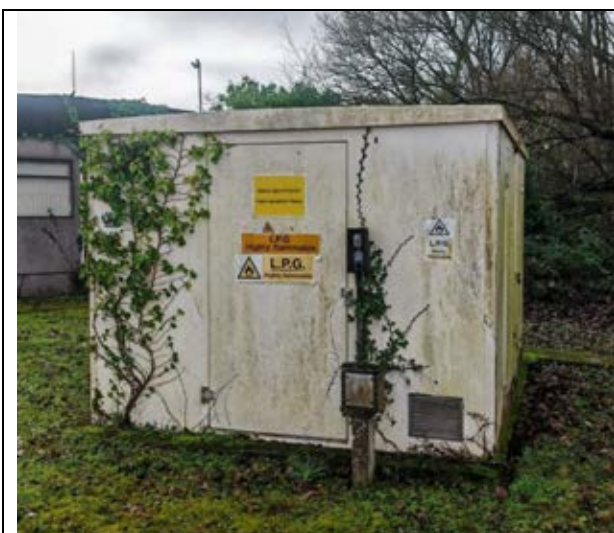
Photo 19: South-eastern elevation and roof junction of B3 showing flat roof structure and fascia detail with minor gaps
