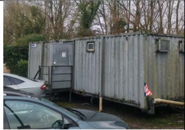
Photo 40: Eastern elevation of B9 showing intact glazing and sealed joints around doors and windows
