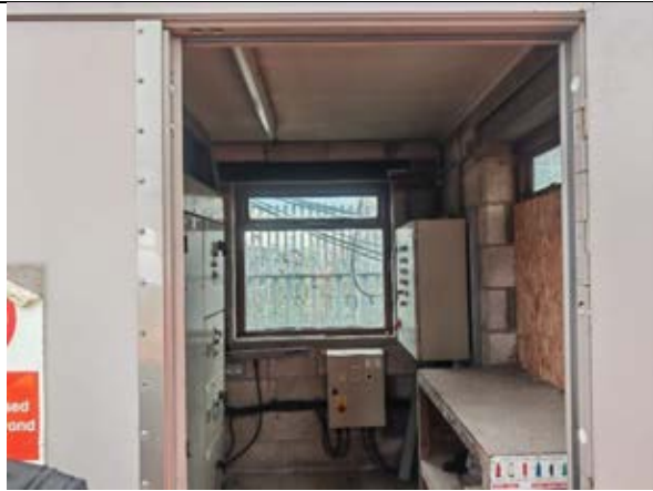
Photo 39: Western elevation of B9 with flat roof and sealed panel construction
