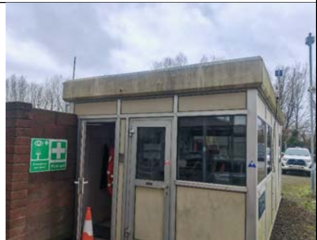
Photo 42: Western elevation of B10 showing large metal-clad walls with minimal gaps or features suitable for bat roosting
