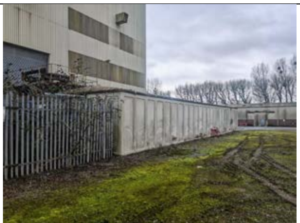
Photo 45: Western elevation of B11 adjacent to B10, showing sealed panel construction with no visible gaps
