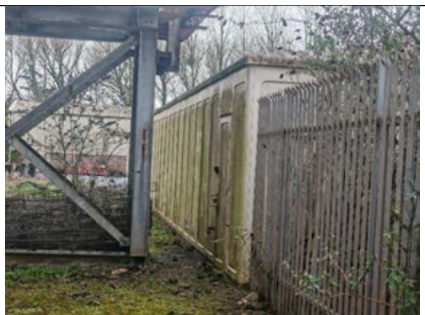
Photo 46: Eastern elevation of B11 showing smooth panel surfaces and tightly fitted doors
