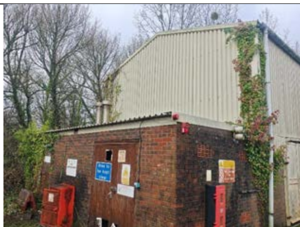
Photo 34: Internal elevation of B6 showing steel frame and roof panels with skylights and suspended crane infrastructure
