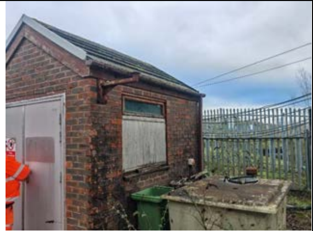
Photo 38: Eastern elevation of B8 raised on supports with sealed panel construction and limited access points
