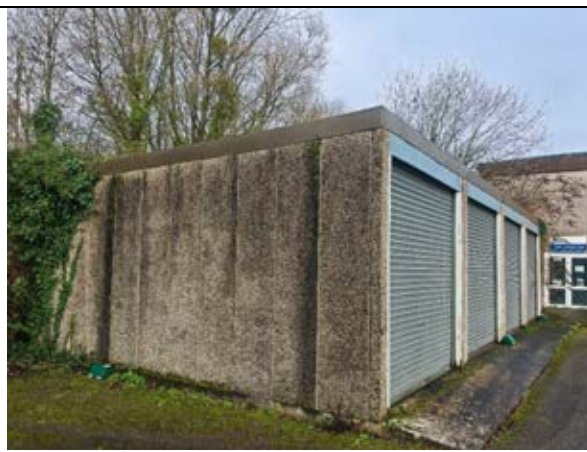
Photo 26: Close-up of roof conduit penetration showing open gap and lifted material forming a crevice suitable for roosting bats
