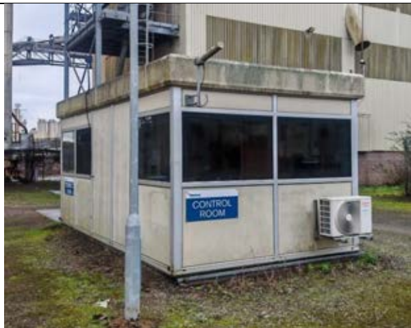
Photo 41: Eastern elevation of B10 showing metal cladding and sealed façade
