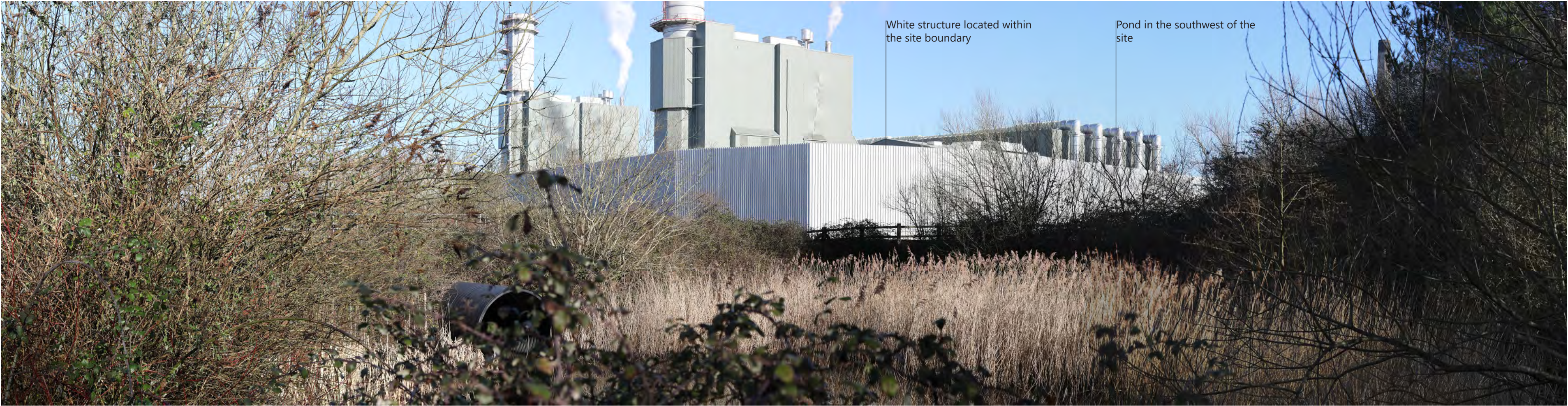
Site photograph 02: View from access path beside the pond to the south of the site, looking northeast
