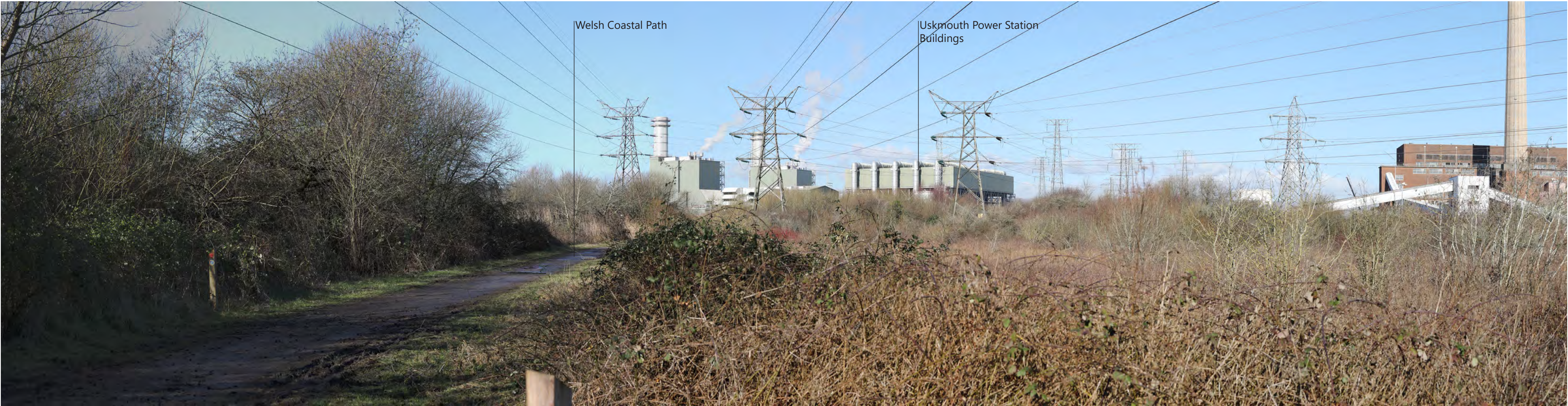
Context View A: Welsh Coastal Path within RSPB Newport Wetlands, looking northwest towards the site
