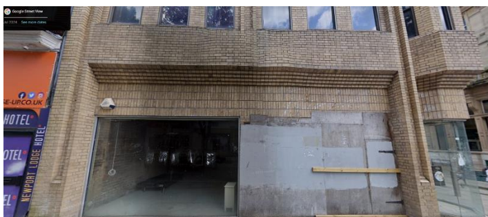
Figure 1 - view of the unit from Commercial St.
