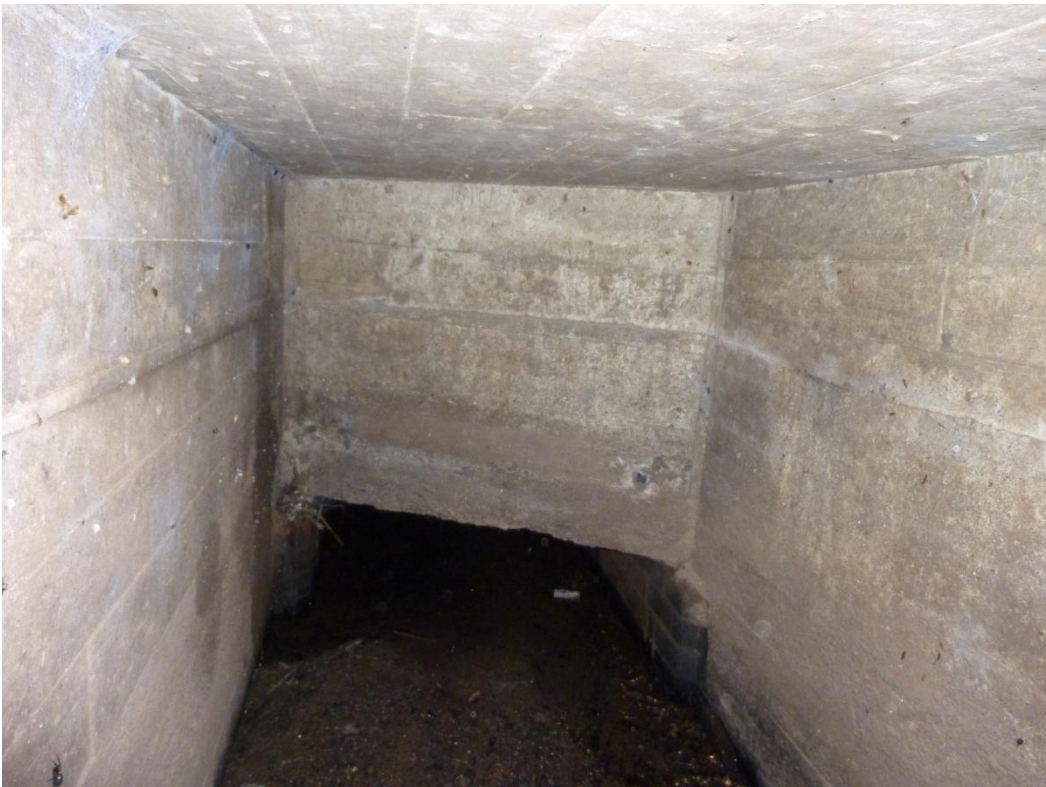
Photo 2 – looking downstream from measurement location (Note severely restricted headroom for passage under roadway)
