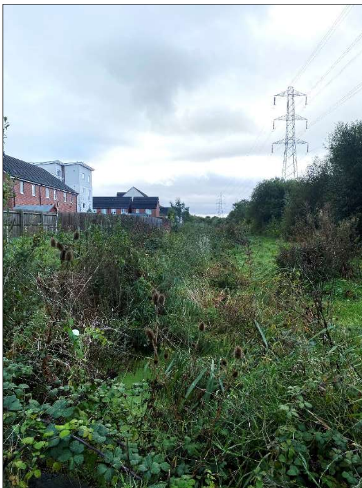
Plate 9. Long ditch Wall, looking south.
