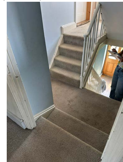
Fig. 19 - First floor landing
