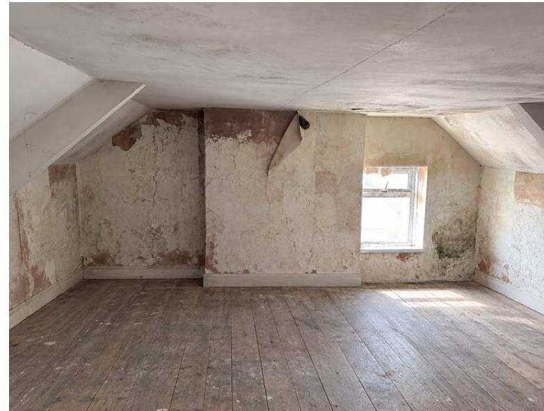
Fig. 14 - Existing second floor bedroom 5
