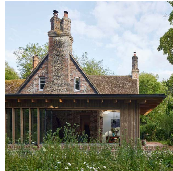
Fig. 31 - Example of contemporary addition to traditional farmhouse
