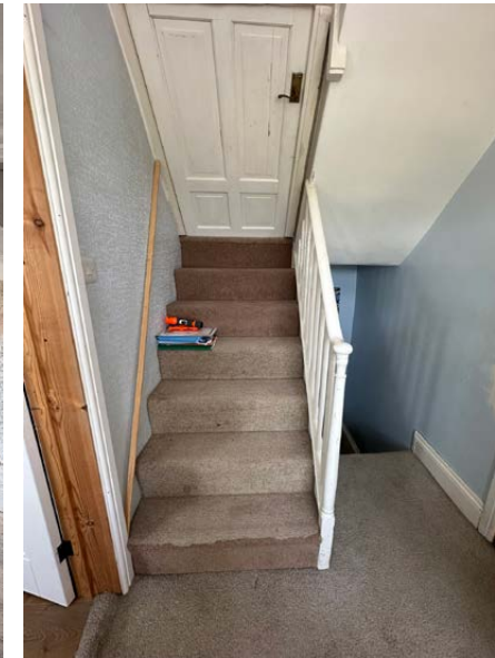
Fig. 15 - Existing stairs to second floor
