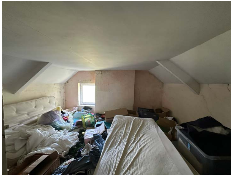
Fig. 13 - Existing second floor bedroom 6
