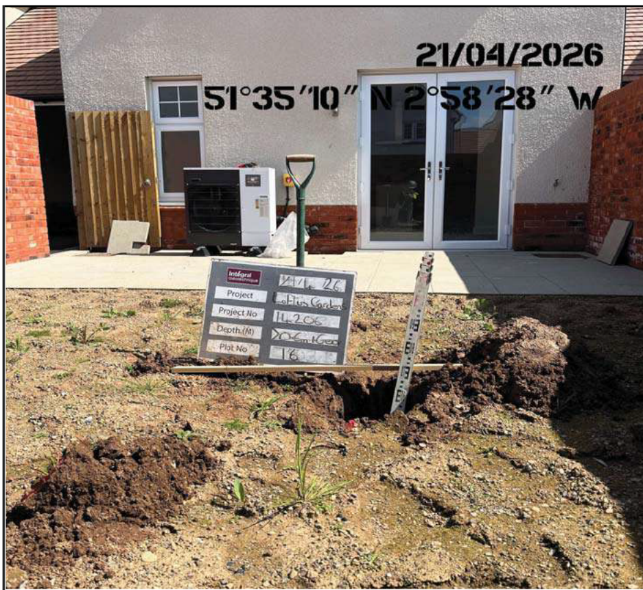
Plot 16 Capping Depth Check Soils
