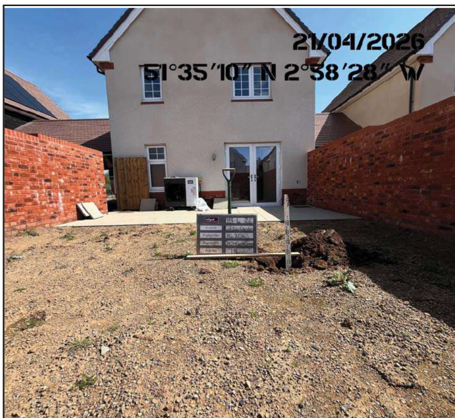
Plot Capping Depth Check Soils
