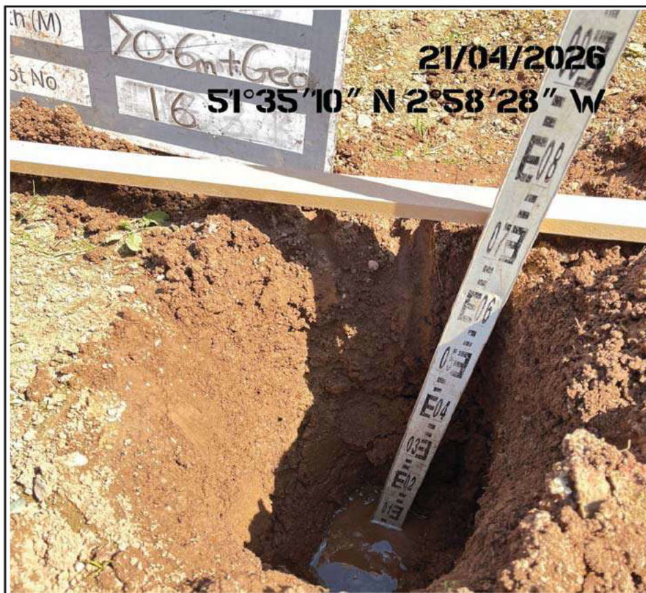
Plot 16 Membrane Placement at Base of Soils
