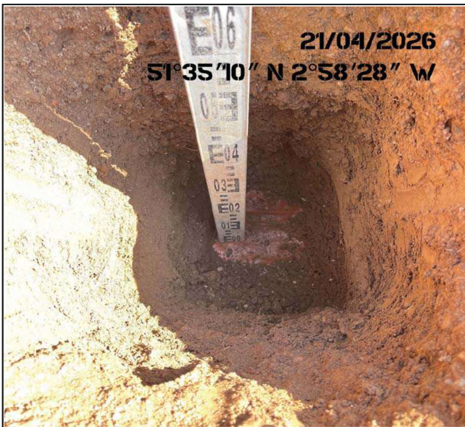
Plot 19 Membrane Placement at Base of Soils
