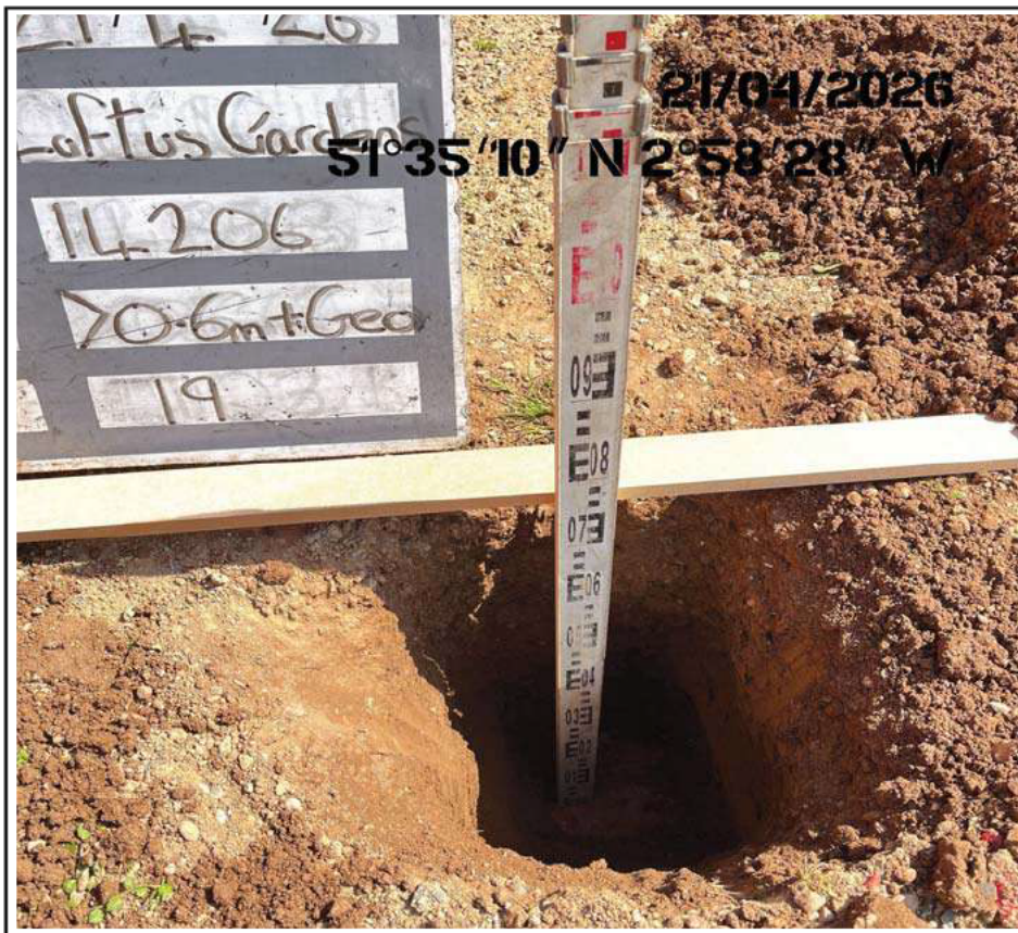
Plot 19 Trial Pit Excavation
