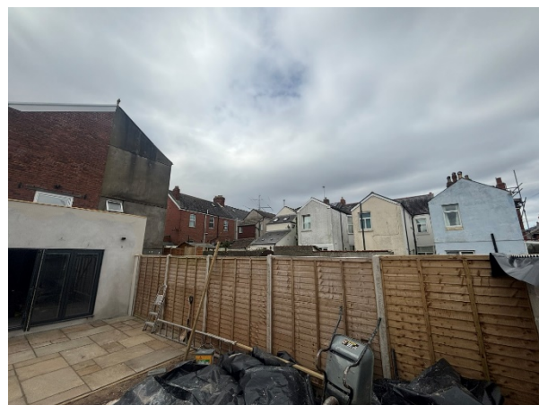
View from window at first floor level over rear extension:
