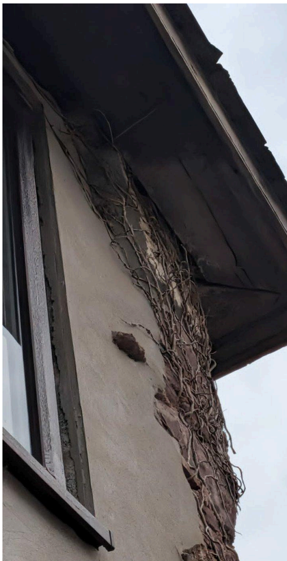
Plate 3 – Eaves and verge detail showing exposed roof timbers, lead flashing and dead climbing vegetation against the rendered wall adjacent to a first-floor window
