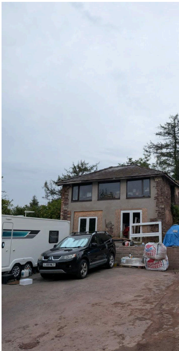
Plate 1 – Front (south-western) elevation showing the rendered first floor over exposed random rubble sandstone, slate hipped roof
