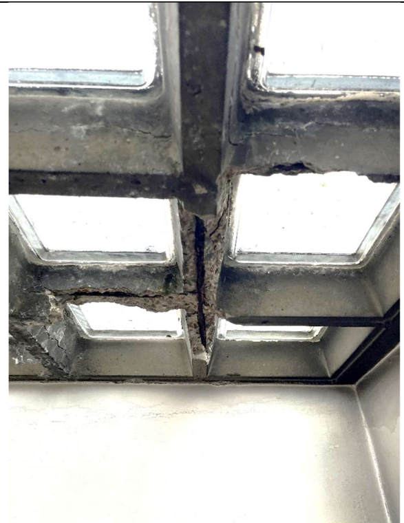
Photo 2. Waffle concrete frame failed
