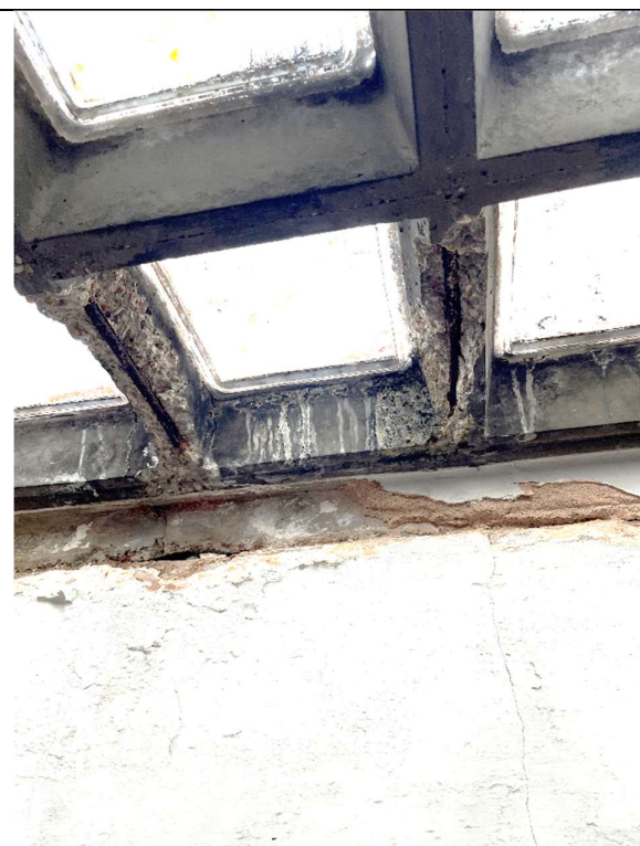
Photo 10. Water ingress, rebar corrosion
