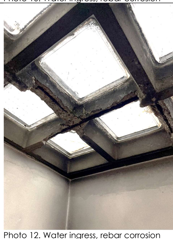
Photo 10. Water ingress, rebar corrosion
