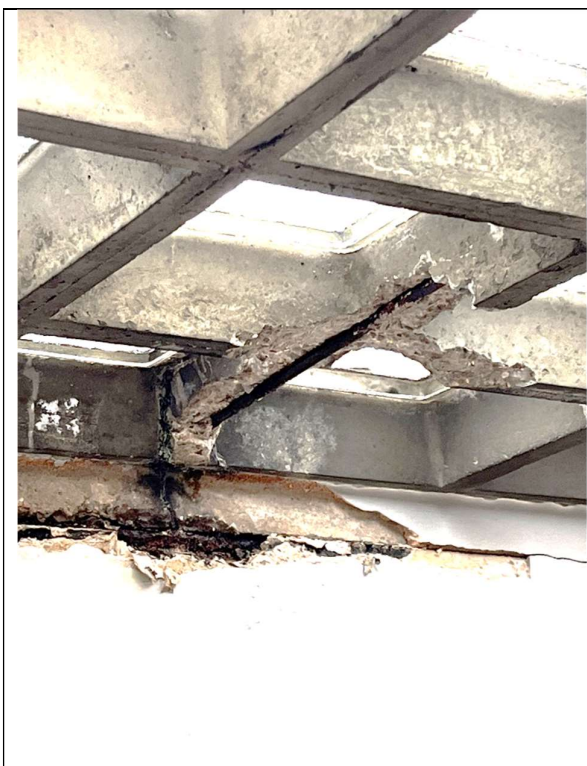
Photo 9. Water ingress, rebar corrosion
