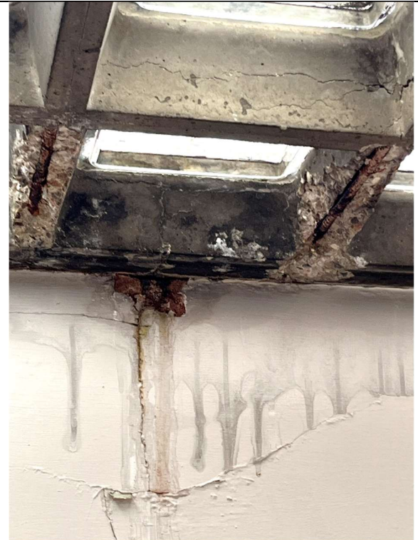
Photo 2. Waffle concrete frame failed
