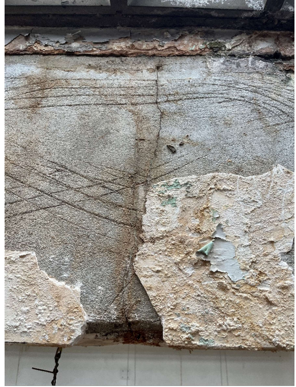
Photo 6. Cracks on beams
