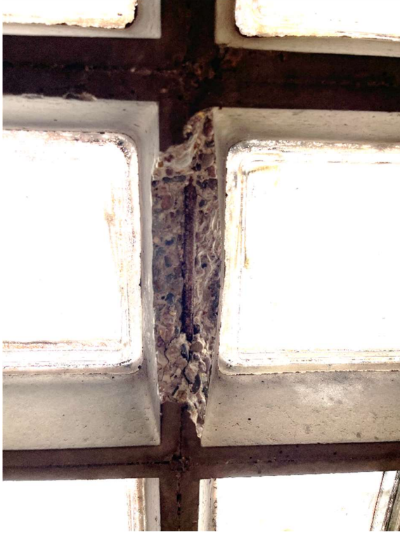
Photo 5. Spalling concrete
