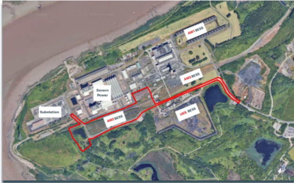
Figure 2: Aerial Image of Proposed BESS Site
