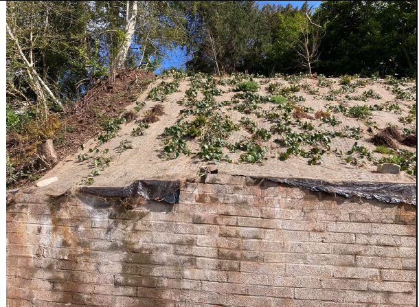
2025 Detail of Greenfix biodegradable matting planted with ivy and ferns
