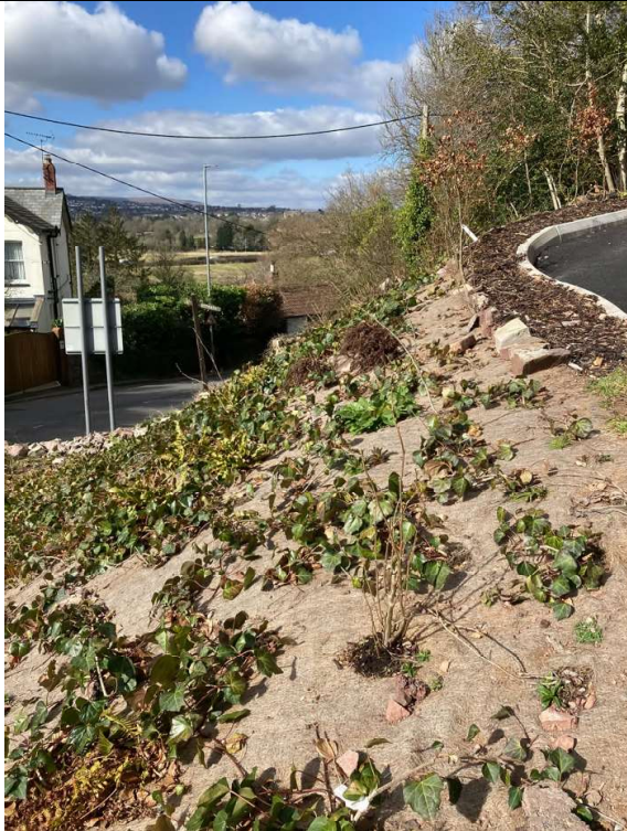
2025 Detail of Greenfix biodegradable matting planted with ivy and ferns [also showing line of hawthorn and hazel]
