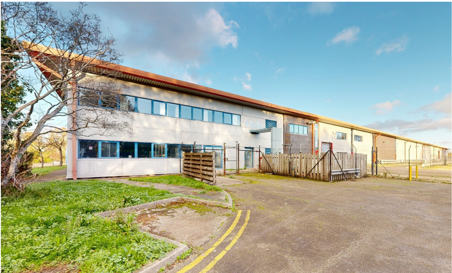
V4- west elevation view of the existing building
