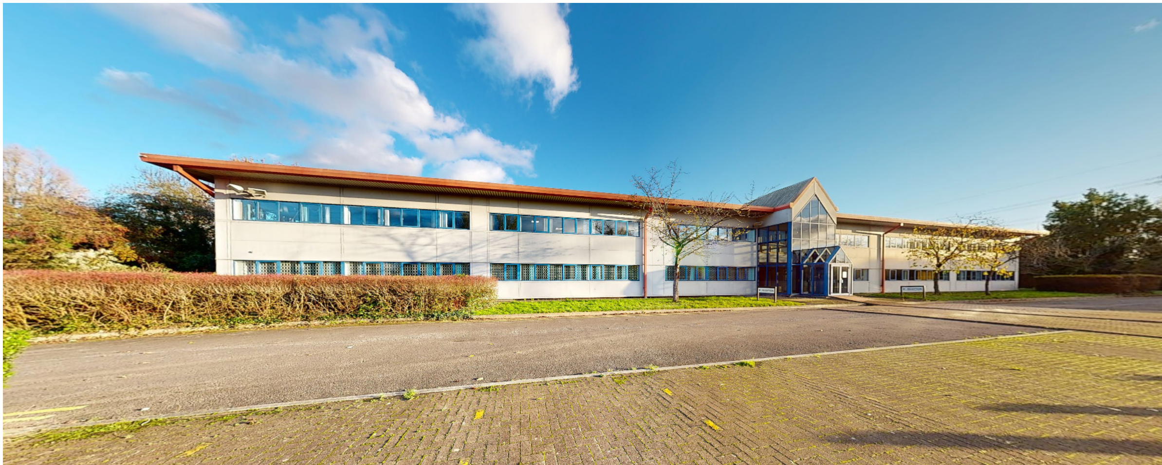
V1- front west elevation view of the existing building
