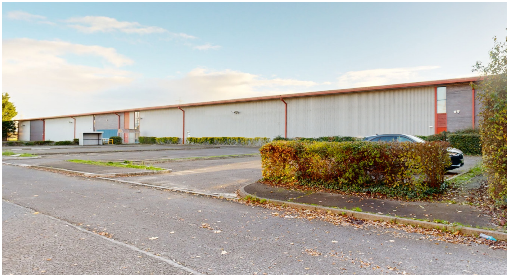
V2- side north elevation view of the existing building
