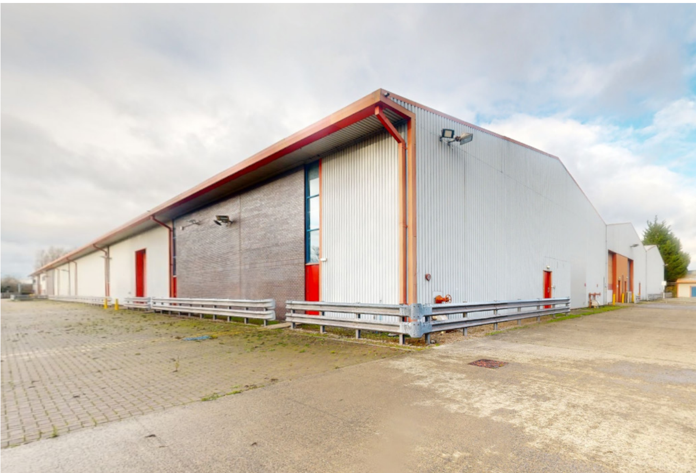
V3- south east and west elevations view of the existing building
