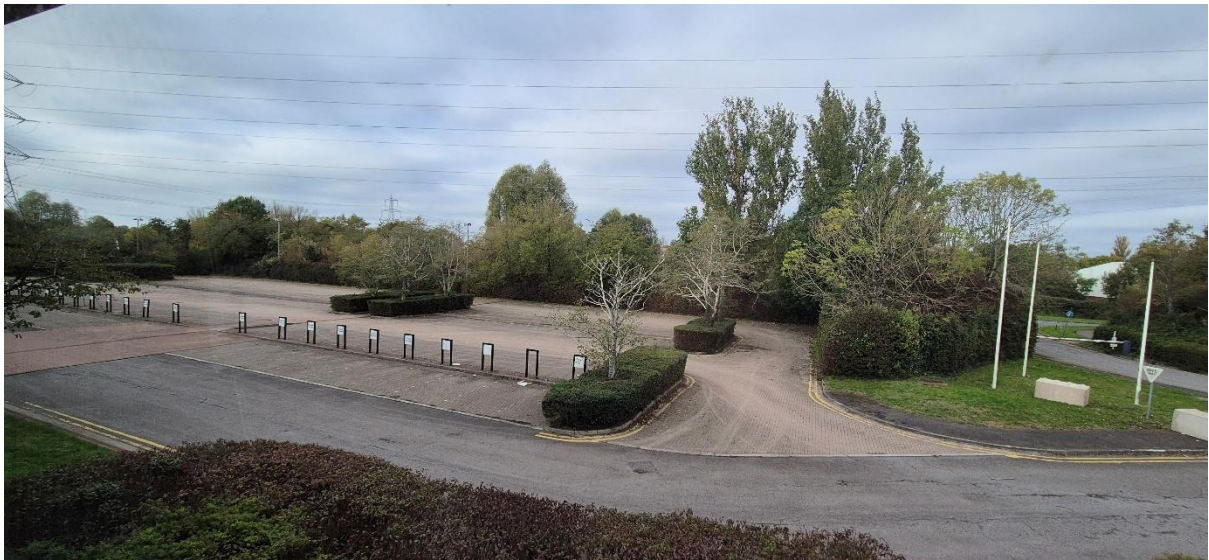
Extensive Frontage Car Park to Western Offices Elevation
