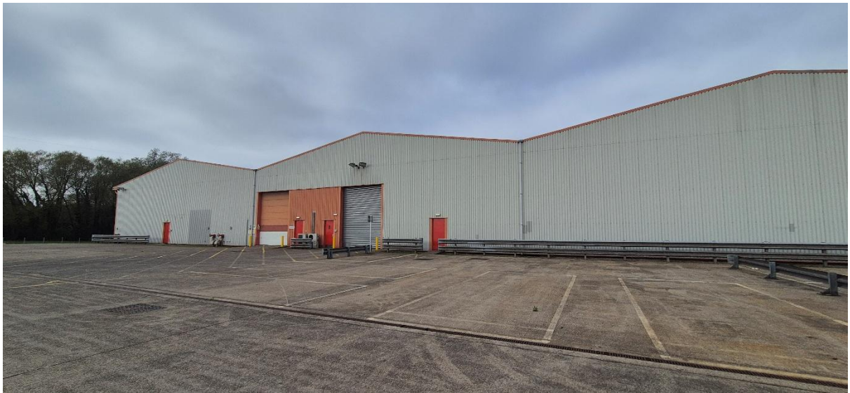
Eastern Warehouse Elevation
