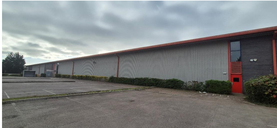
View of Existing Building – Northern Elevation
