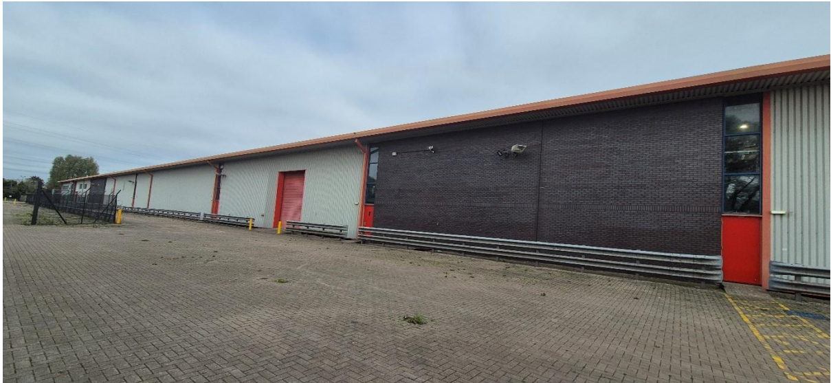
Warehouse Southern Elevation
