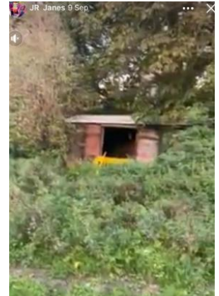
A photo of the site (see right) that shows an old small stable building / shed
