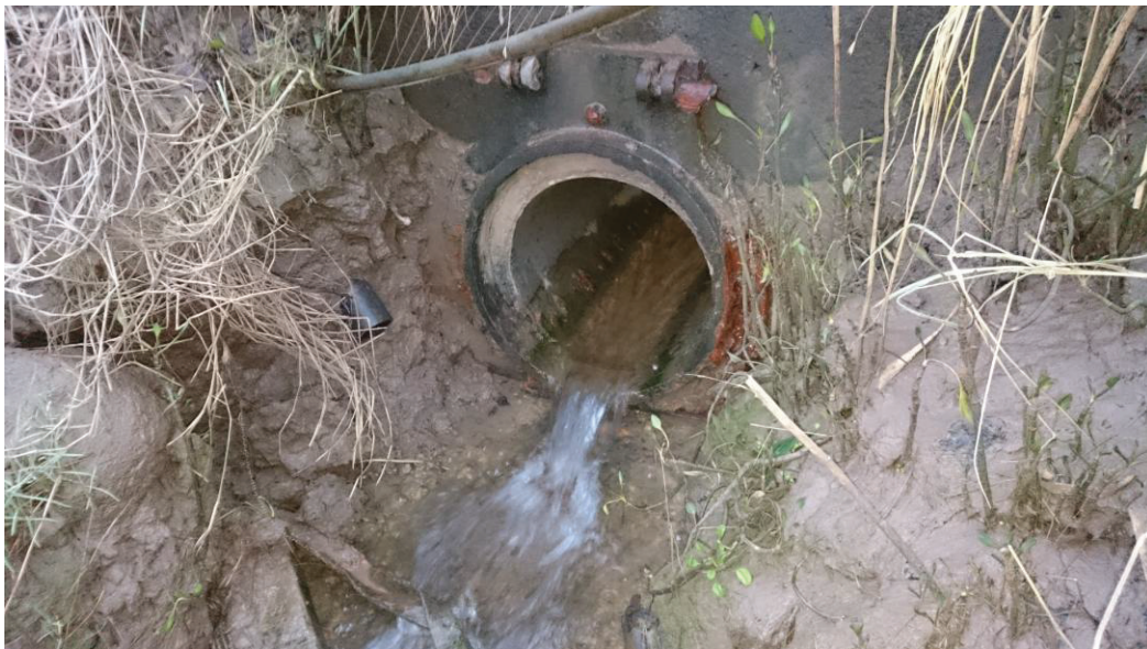
Photo 2-existing tidal flap in headwall
