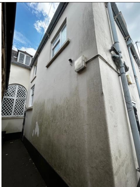
Rear elevation – Access to stairwell
