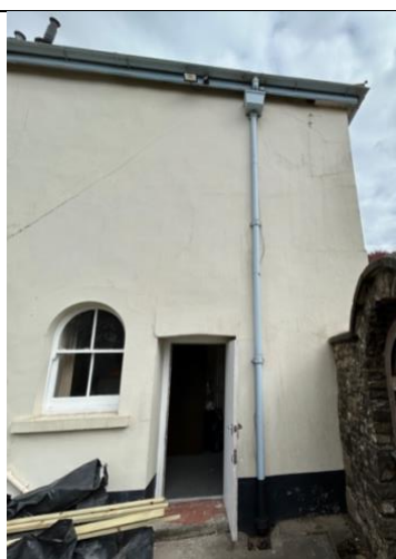
Side elevation – trustees office and door
