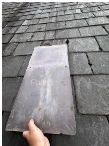
Courtyard roof – (left slope) Salvaged Penrhyn
