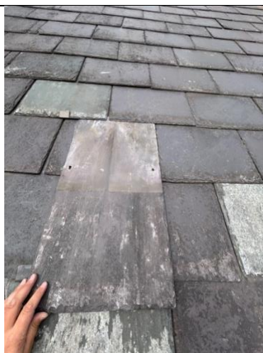
Courtyard roof – Salvaged Penrhyn
