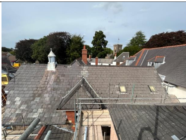
Courtyard roof – Right slope (when facing gable from courtyard) – Welsh slate (various) and man-made slates various widths
