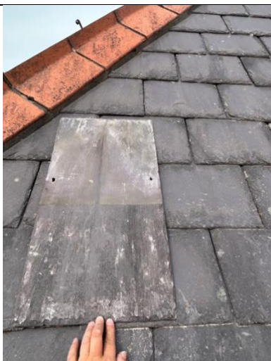
Schoolhouse roof – Salvaged Penrhyn
