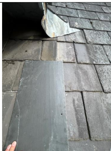
Courtyard roof – front slope rear dormer - Glendyne 250 x 500
