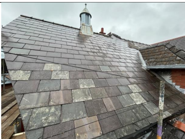
Courtyard roof – Right slope - 07.08.25 – Wet conditions Various size slates – larger welsh
