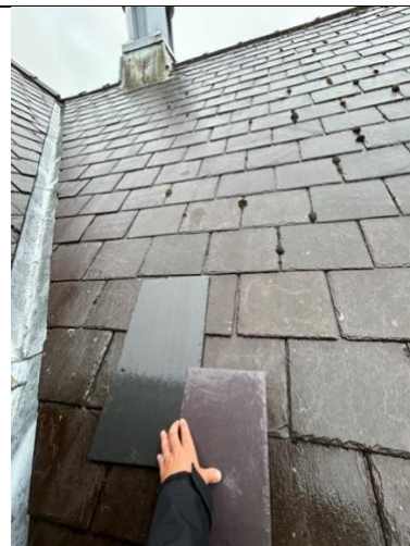
Courtyard roof – (left slope) 07.08.25 Wet conditions – NEW Glendyne and NEW penrhyn
