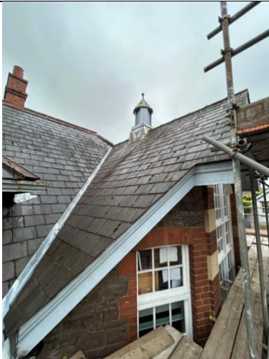
Courtyard roof – (left slope) 07.08.25 Wet conditions
