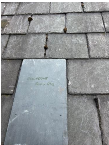
Courtyard roof – (left slope) Glendyne 250 x 500 (size match – to all other roof areas over courtyard)
