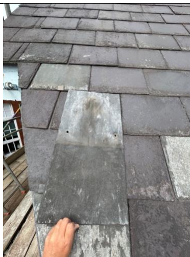
Courtyard roof – Salvaged Welsh grey
