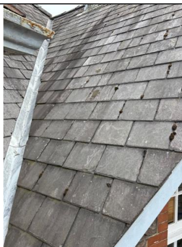
Courtyard roof – (left slope) 06.08.25 dry conditions
