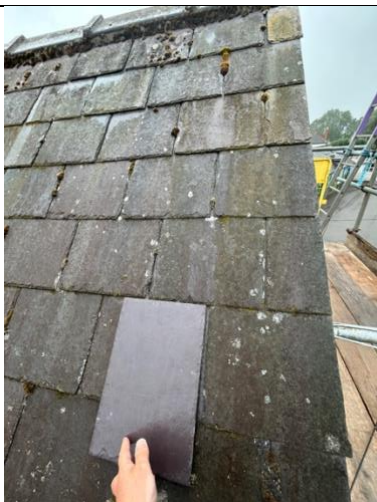
Courtyard roof – (left slope) 07.08.25 Wet conditions – NEW penrhyn
