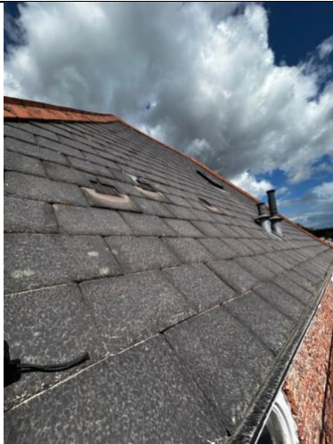
Main school roof adjacent pyramid
