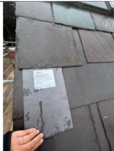
Courtyard roof – (right slope) 07.08.25 Wet conditions – NEW penrhyn
