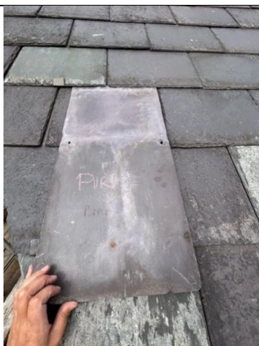
Courtyard roof – Salvaged Penrhyn
