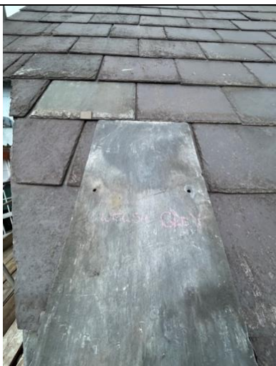
Courtyard roof – Salvaged Welsh grey
