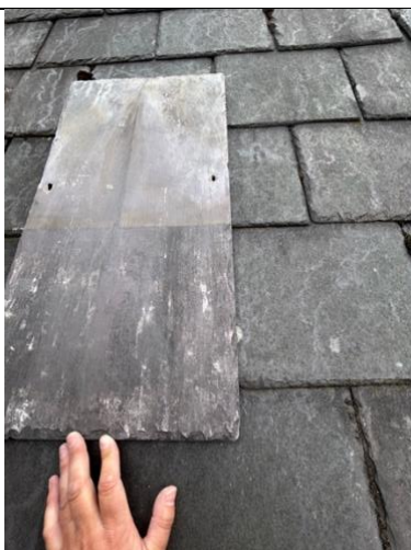
Courtyard roof – (left slope) Salvaged Penrhyn
