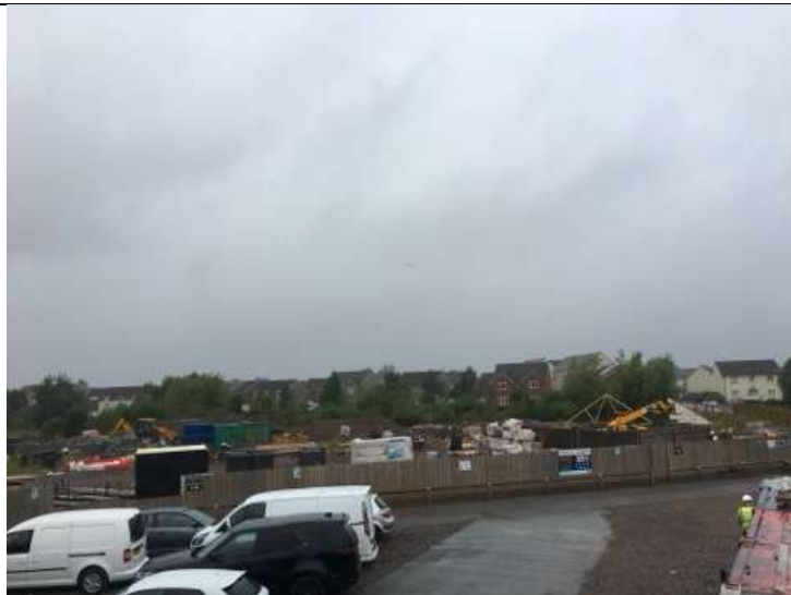
Photo 7: View towards West from St Modwen's site office 8 th August 2024.
