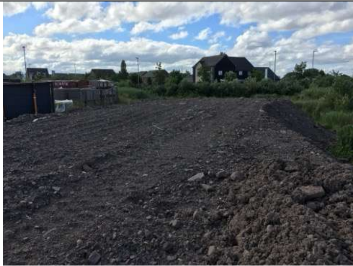
Photo 6: View towards South from South of the site 10 th June 2024.
